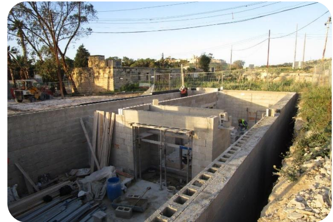
Construction Works at Ta' Qali Crafts Village
