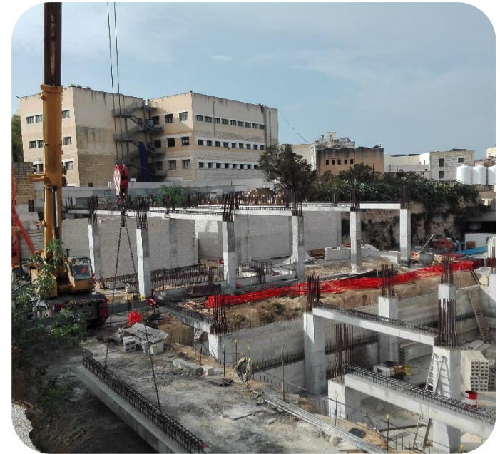
Ongoing works at the Institute of Engineering and Transport (IET) – MCAST
