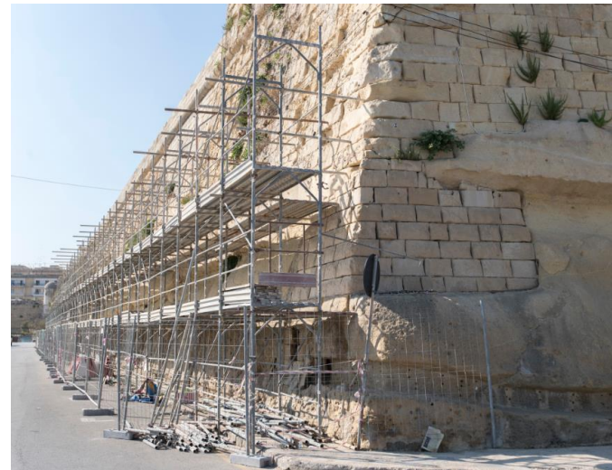
Restoration of St Sebastian and English Curtain
