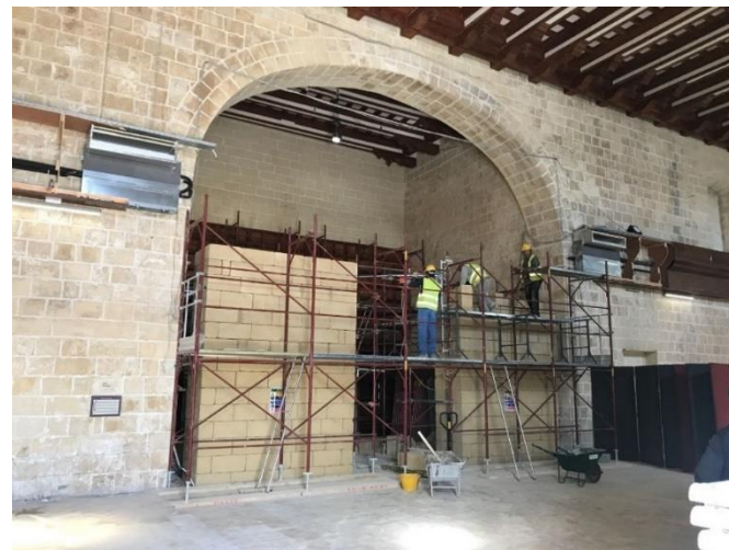
Works being carried out at MCC
