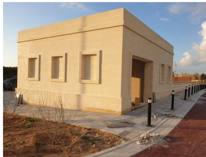
Construction works - Ta' Qali Crafts Village
