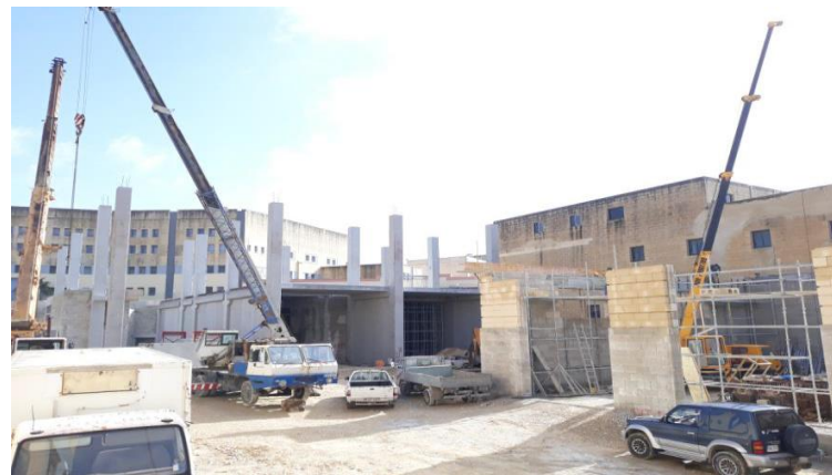
Works at Xewkija Industrial Park (Tal Hofra)
