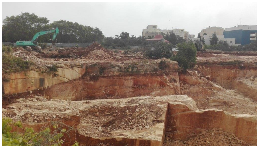
Excavation works in relation to SLC
