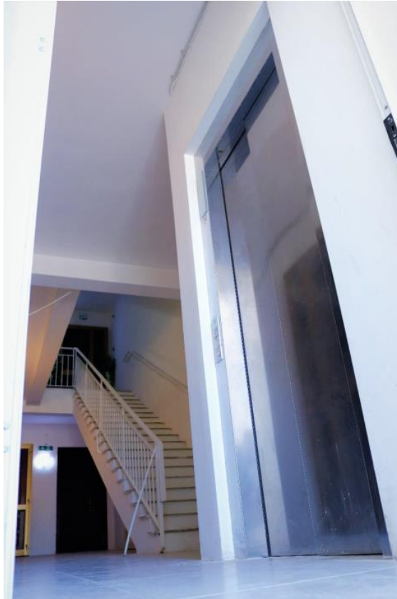
Social Housing Estates upgrade with lift retrofitting
