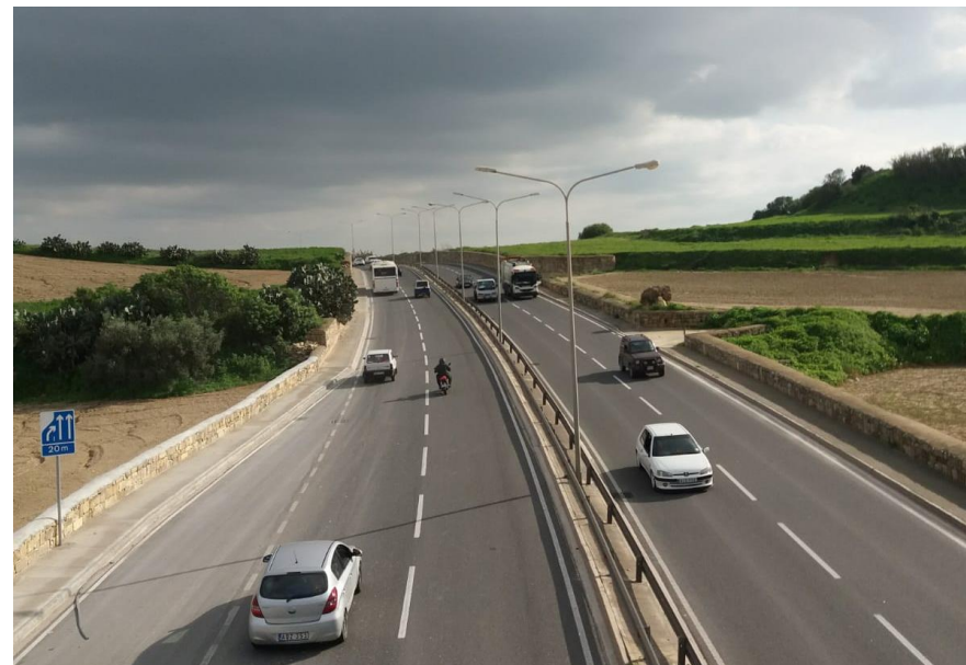
Retrofitting of Streetlighting
