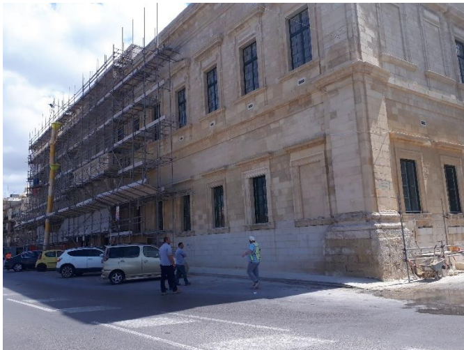
Restoration of Auberge de Baviere Façade
