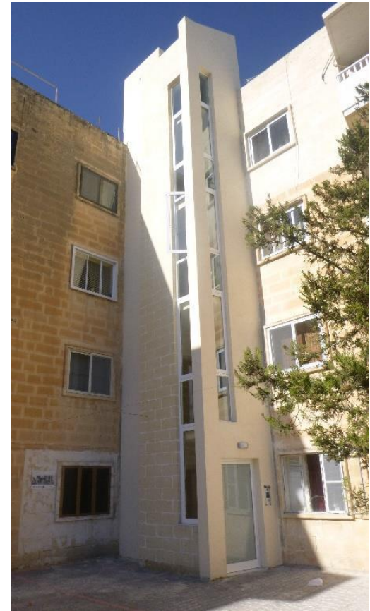
Social Housing - Installation of energy efficient lifts
