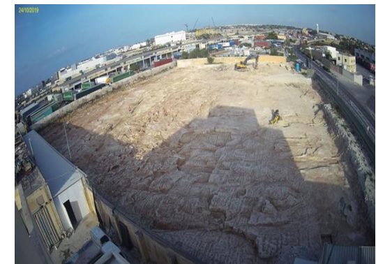
MMRF ongoing excavations
