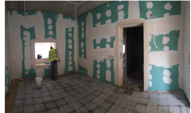
Rehabilitation works for social housing
