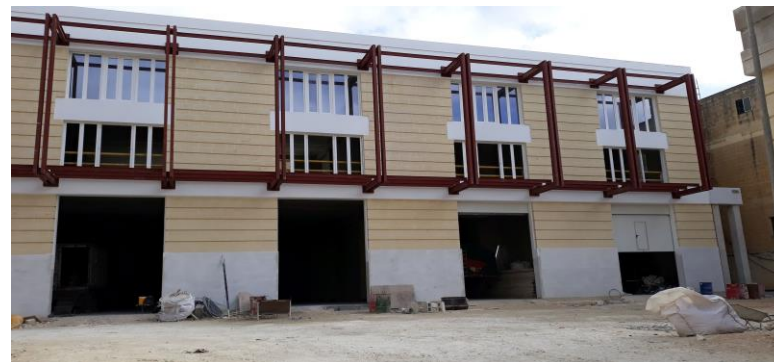
Industrial Workshop Complex, Xewkija
