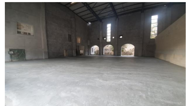
Civil works at Gozo RO
