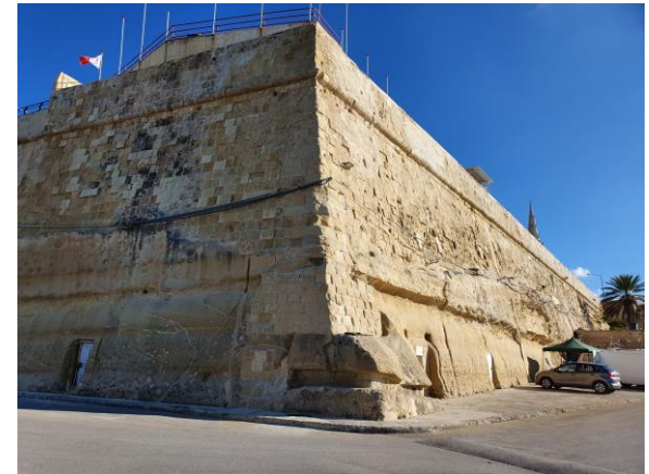
Restoration of Valletta fortifications
