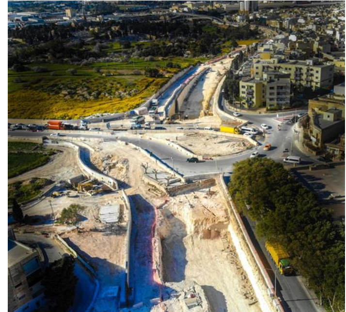
Ongoing works on the Santa Lucija Underpass
