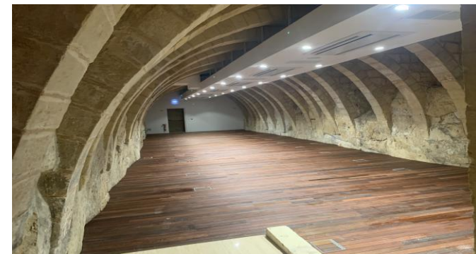
Restoration – Tank rooms at MCC
