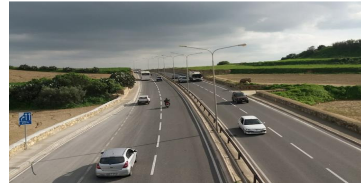
Retrofitting of street lighting
