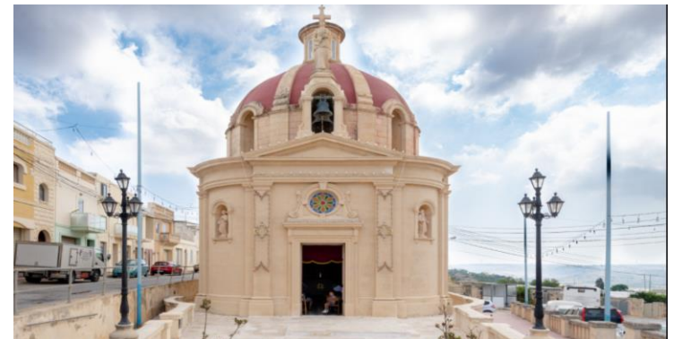
Restoration of Bidnija Church
