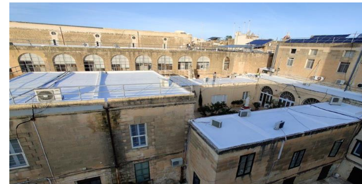
Roof insulation at the Gozo Administration Centre
