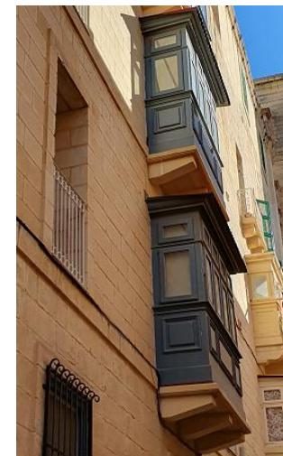
Restoration of Maltese balconies - Valletta
