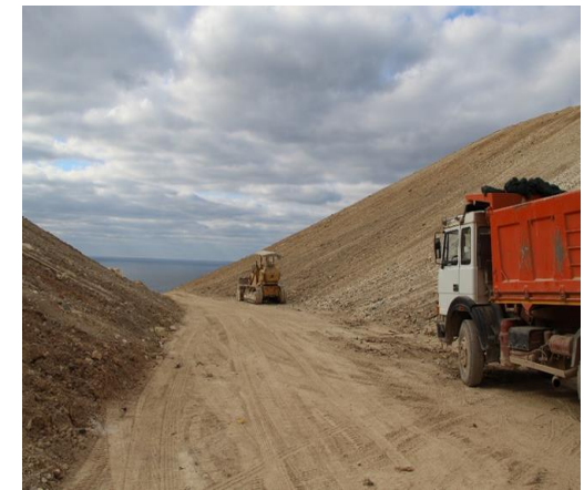
Wied Fulija rehabilitation works
