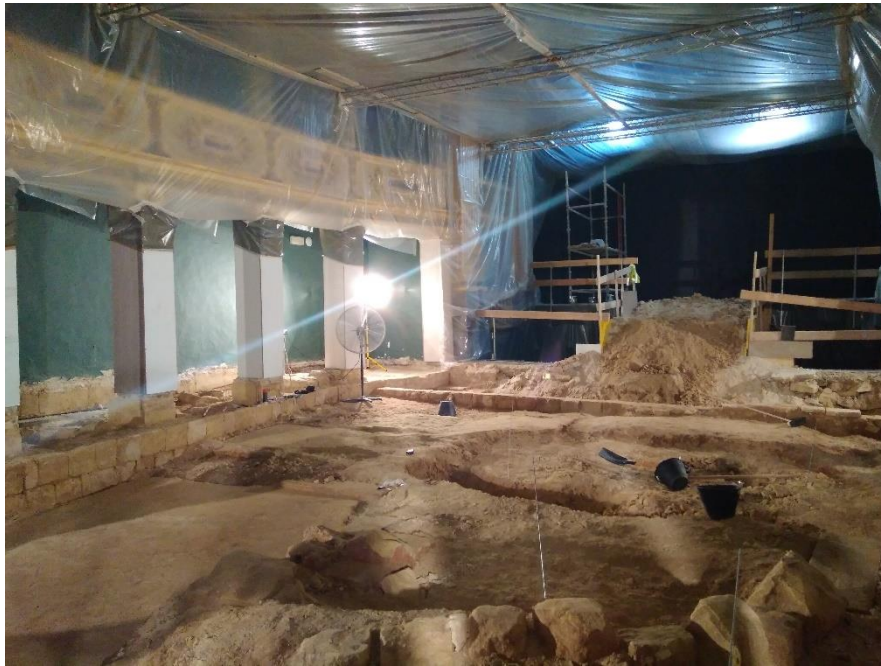
Ongoing works at the Manoel Theatre
