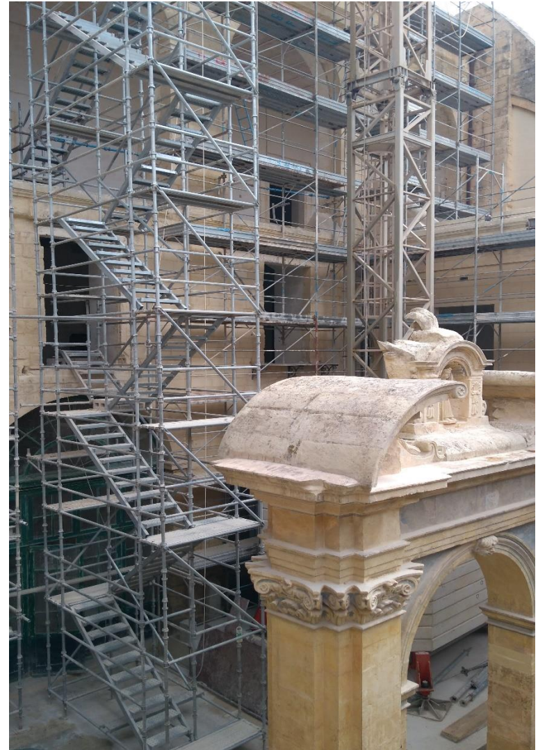
Scaffolding on site at the MUZA building
