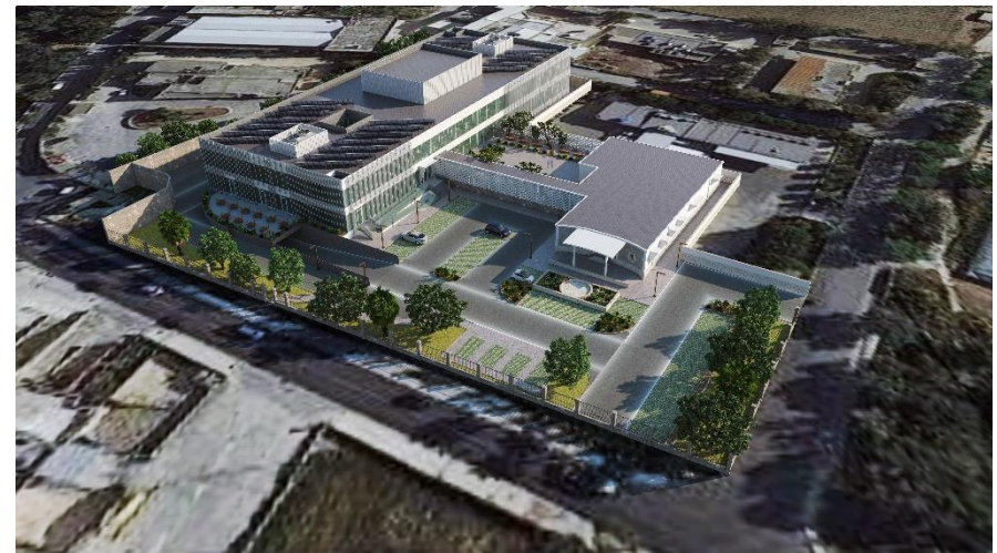
Enterprise Hub in Xewkija (ex-Malta Dairy Products building)
