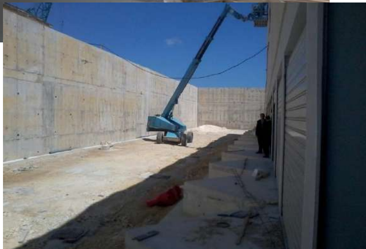
Images nos.7-8 [above]: Construction works at the new fish market.
