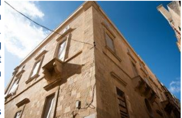
Upgrading of 90, West Street
