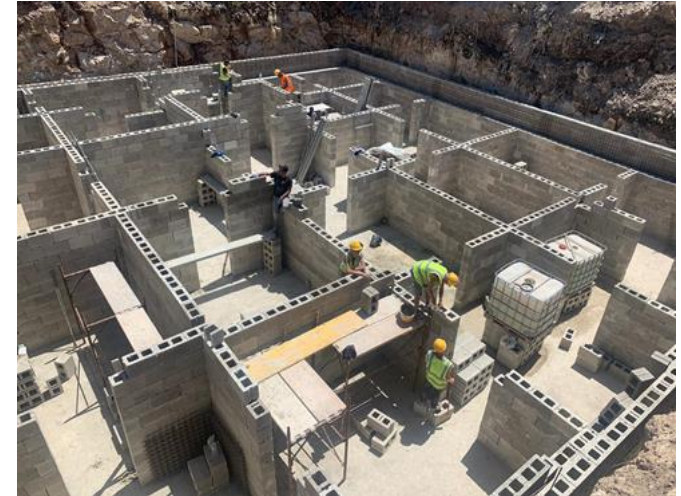
Construction of reservoir at Wied Fulija landfill site
