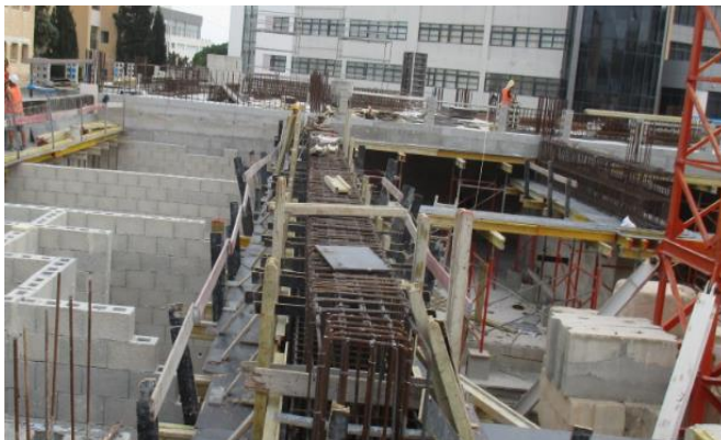
Ongoing construction works at the IICT
