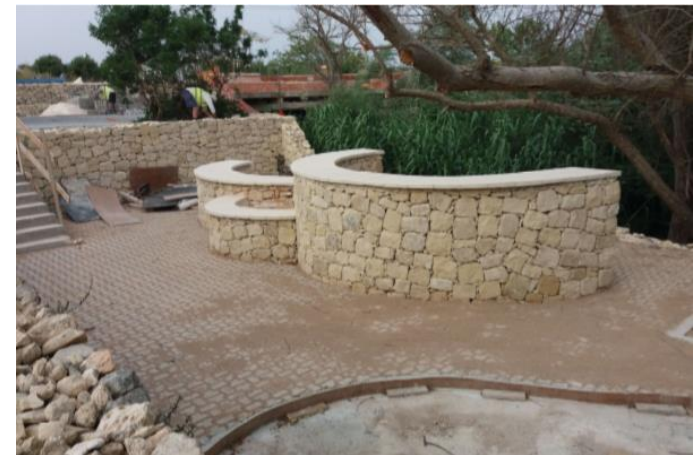
Ongoing works at the Family Park at Chadwick Lakes
