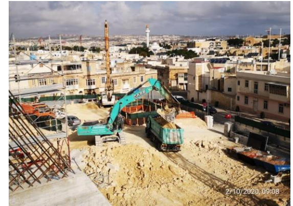
Paola Regional Hub - excavation works
