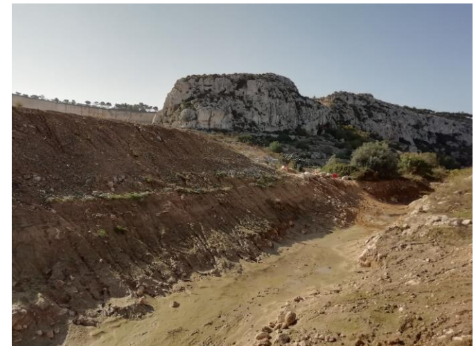
Basin excavation works under the RainWiin pilot project
