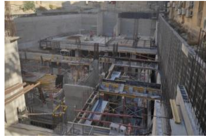
Construction works at TRAKE's main building
