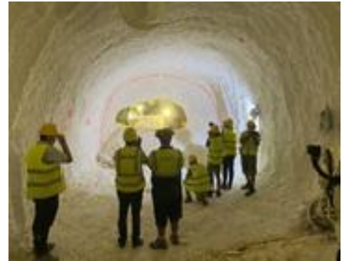
Water Major Project: Iklin-Ibraġġ breakthrough
