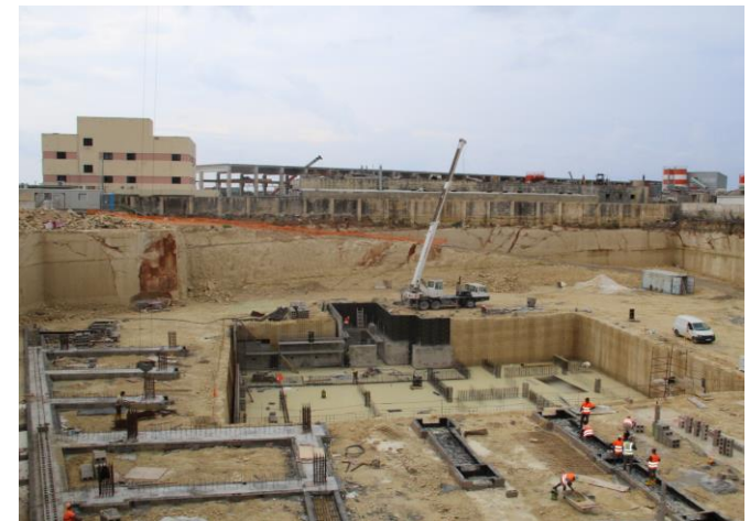
Construction of foundations at the MMRF site
