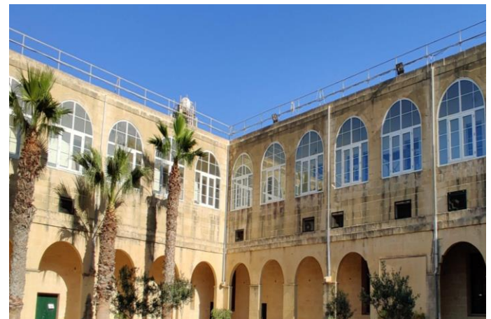
Double-glazing apertures installed at the Gozo Administration Centre
