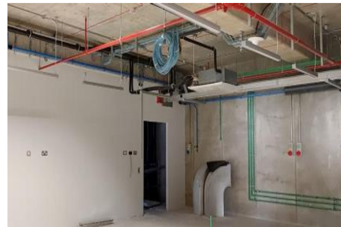
Ongoing works at MMEL – Level -1
