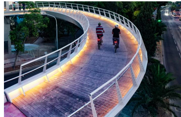
The completed Pedestrian Bridge at Blata I-Bajda
