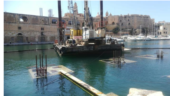
Ongoing works at the Bormla ferry landing site
