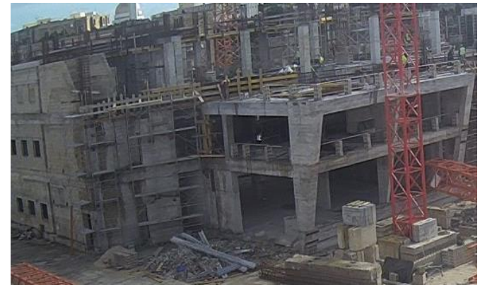
Advanced construction works at the Resource Centre
