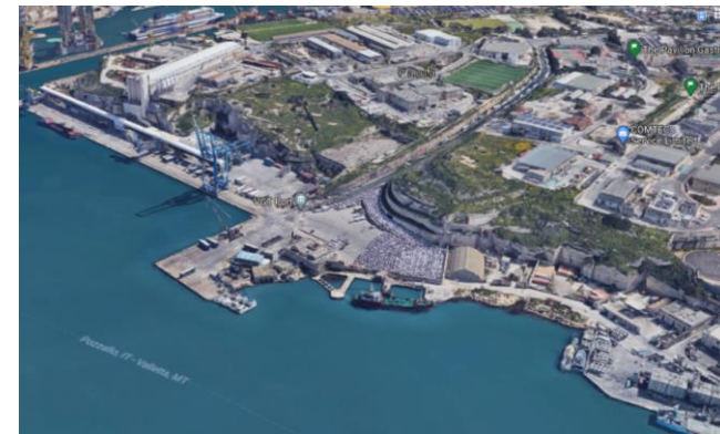
Site of new cargo facility
