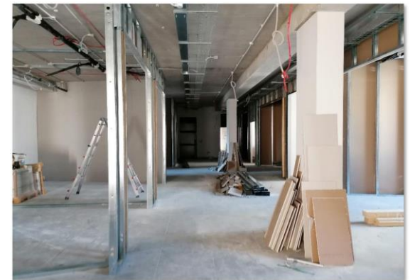
Caritas Community Centre - M&E and Finishes works
