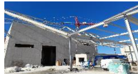
Ongoing construction works at the MMRF site
