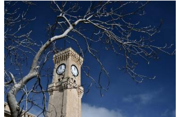
Ongoing restoration works at Mtarfa's historic clock tower
