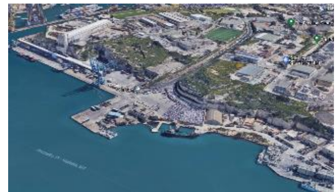
Site of new cargo facility
