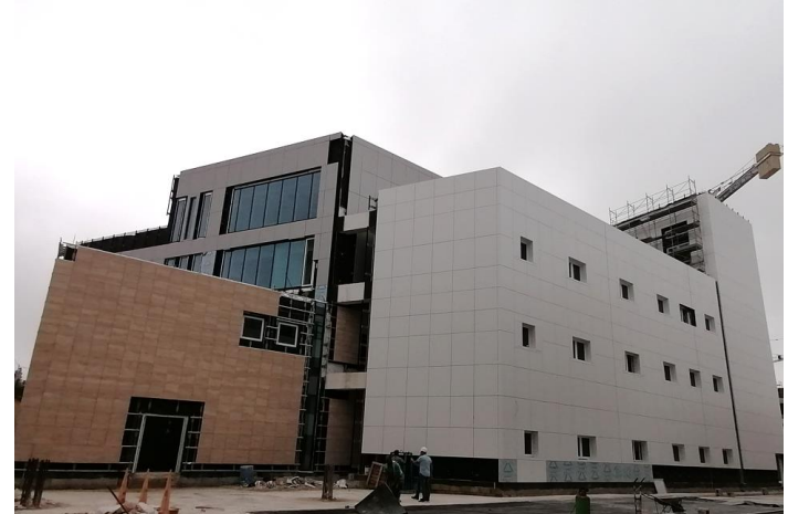
Ongoing finishing works at MRC - MCAST
