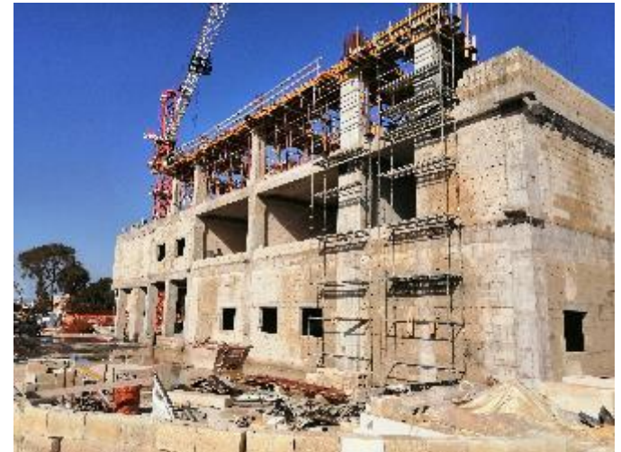
MCAST construction works at IICT site
