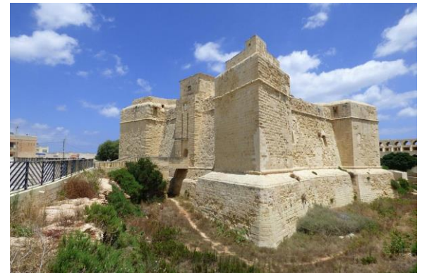
Ongoing restoration works at St Thomas Tower in Marsaskala
