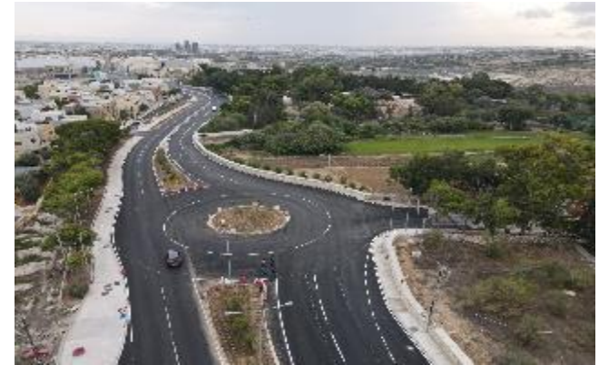
TEN-T Road Infrastructure: Works on Mrieħel – Ta' Srina
