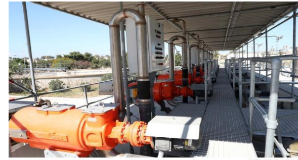
'Moving Bed Biological Reactor' installed at Sant'Antnin wastewater treatment plant
