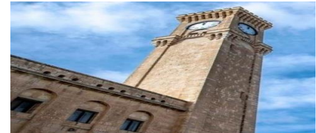
Restoration works at Mtarfa's historic clock tower
