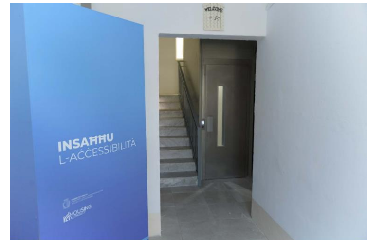
Installation of new lifts at San Ġwann Social Housing Estate
