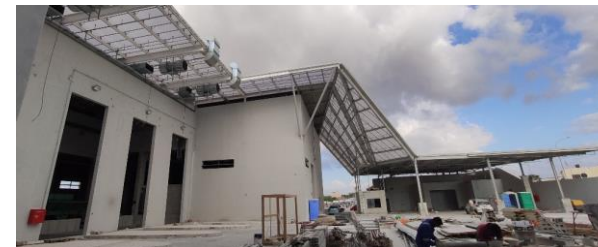
Ongoing civil works at the MMRF site
