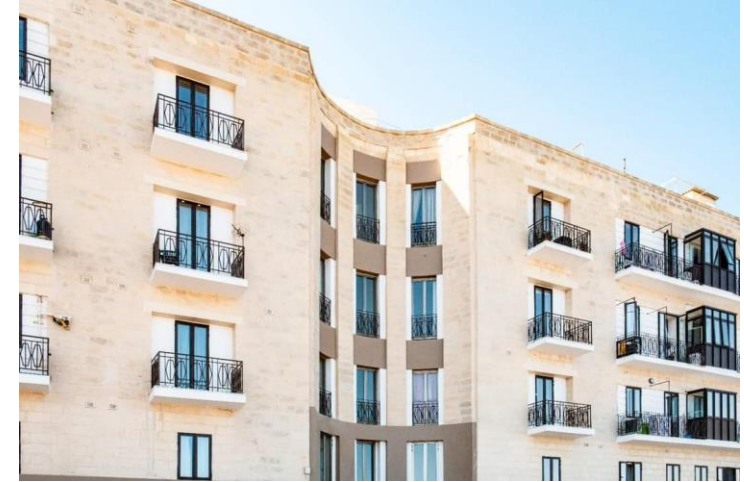
Restoration of one apartment façade at Mattia Preti square.
