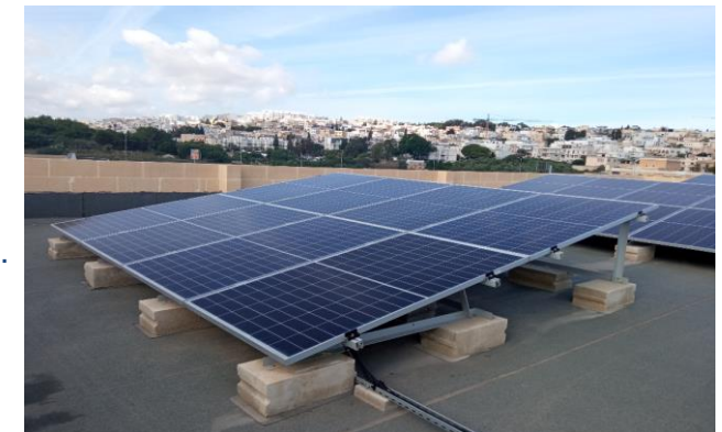
Installation of PV panels - St. Monica School, Gzira
