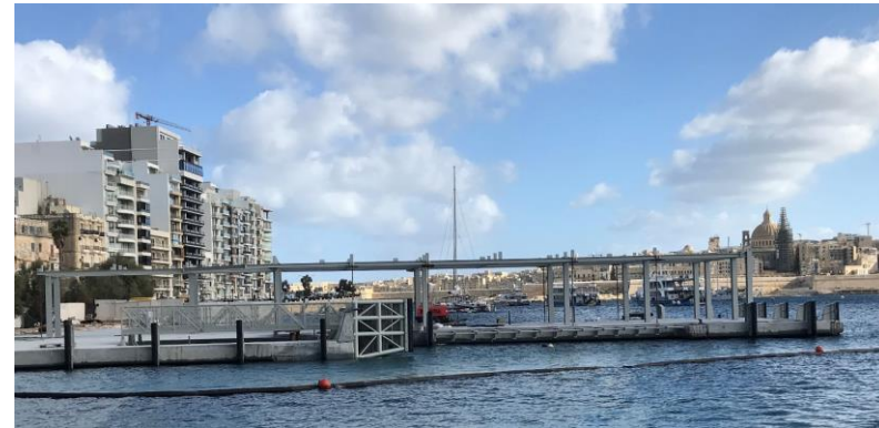
Ongoing works at Sliema Ferry Landing
