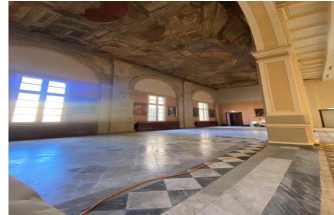
Restoration works on the Piano Nobile corridors at the Grandmasters' Palace.
