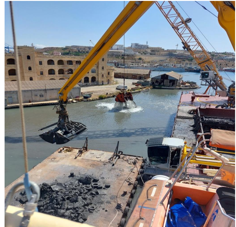
Dredging works in the Grand Harbour
