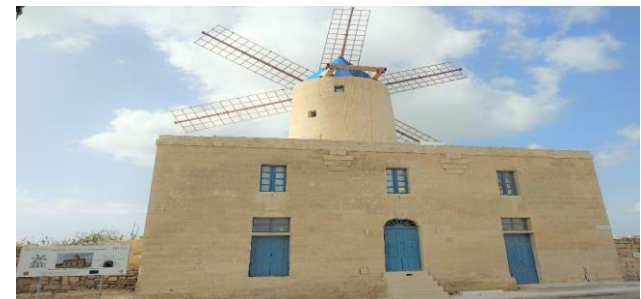
Ongoing restoration works at Culture Mill
