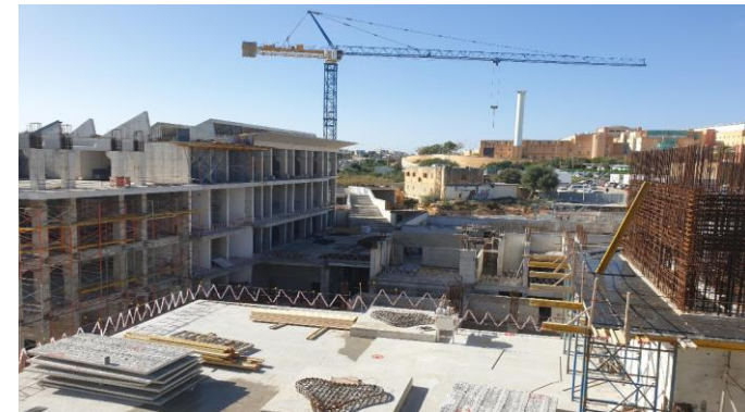
Construction works at SLC site at the University of Malta campus
