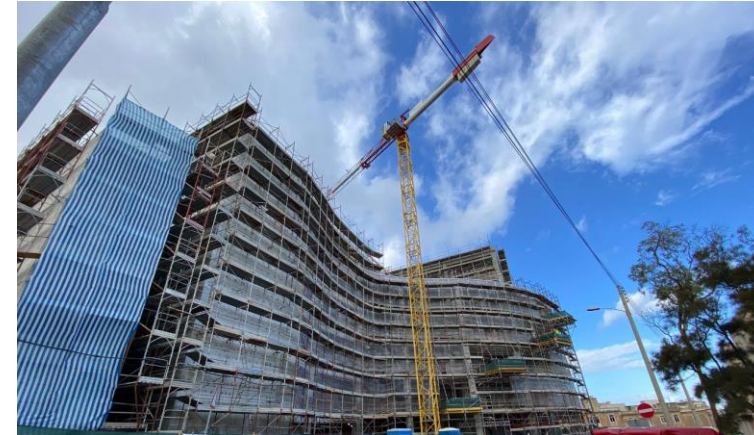
Construction works at Paola Regional Hub Primary Health Care Centre
