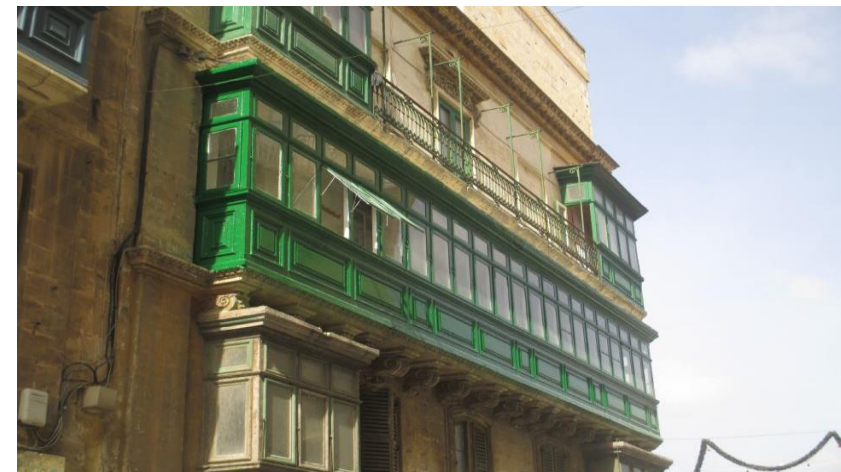
Restoration works under the Marsamxett Balconies Scheme
