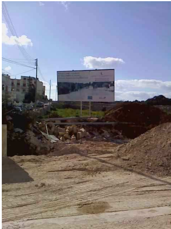
Figure 2 - ERDF 048 – Works being undertaken within Phase 5 of Marsascala Road
