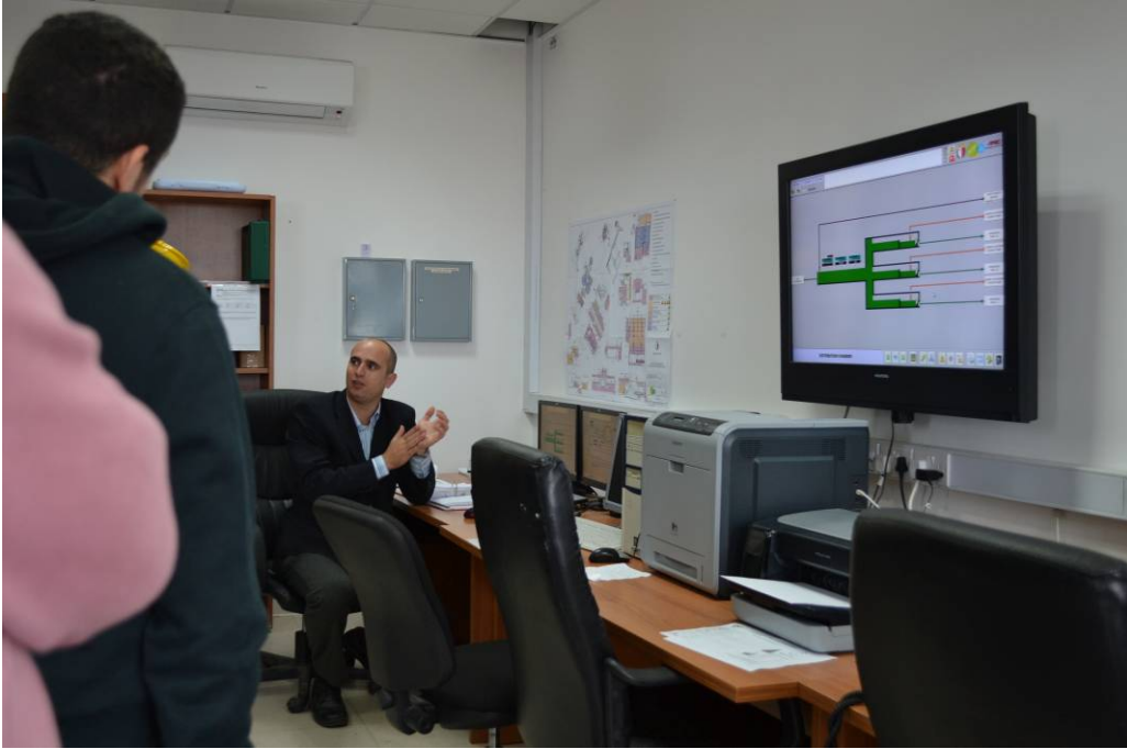
Figure 6.1 CF 116 Project Leader explaining the 'behind the scenes' work at the Malta South Sewage Treatment Plant
