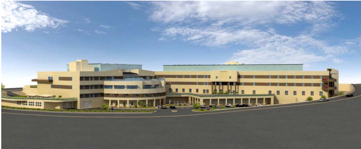
Figure 4.2 – Mater Dei Hospital Oncology Centre
