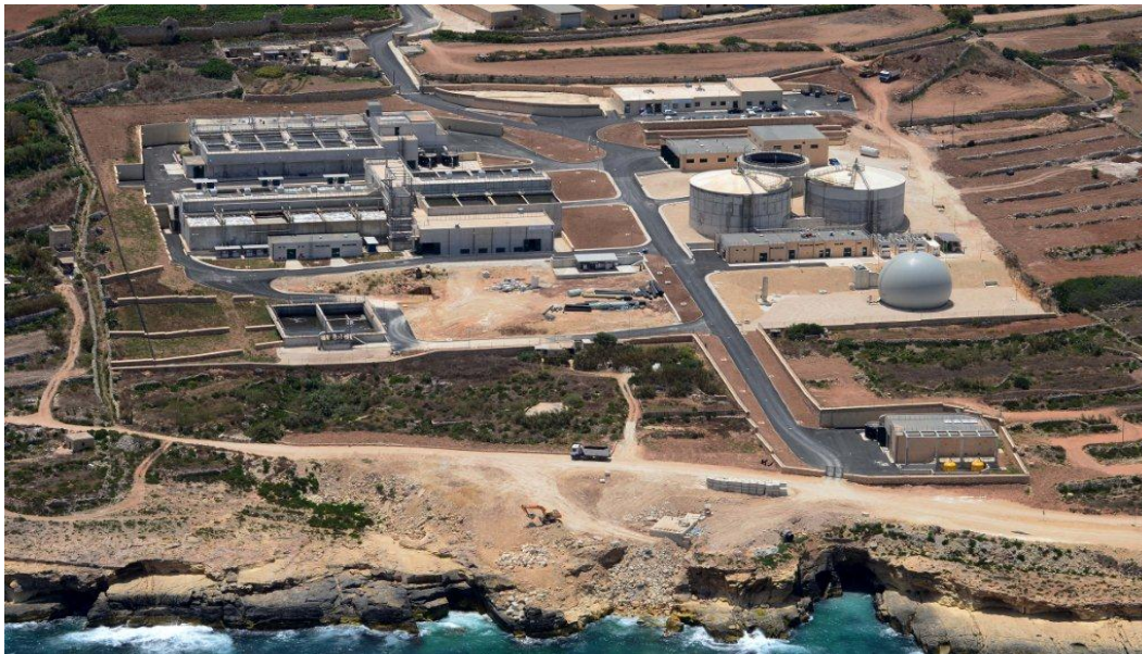
Figure 4.1 – Urban Wastewater Treatment Plant
