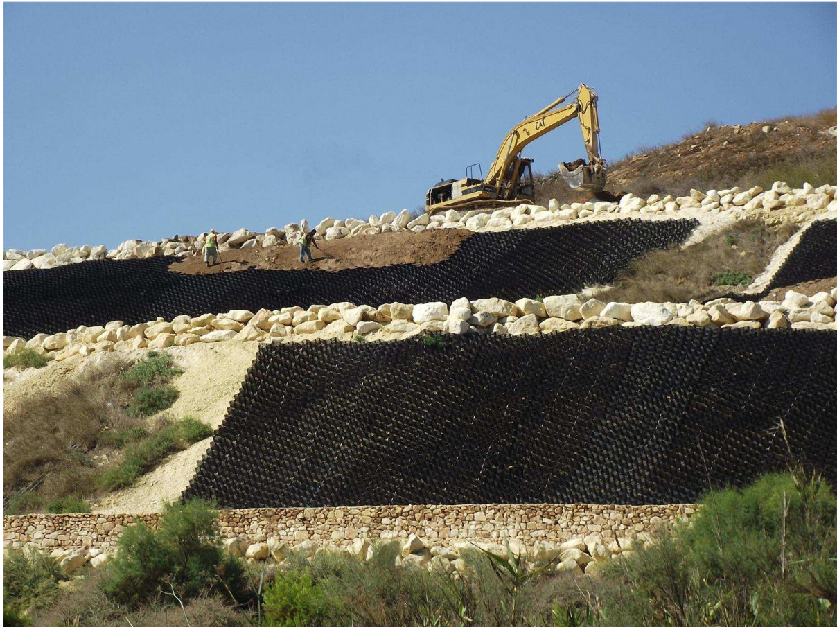
Figure - Ongoing works at the Maghtab landfill
