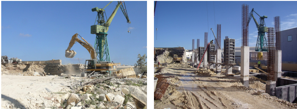
Figure 4: Demolition and Construction of the New Fish Market
