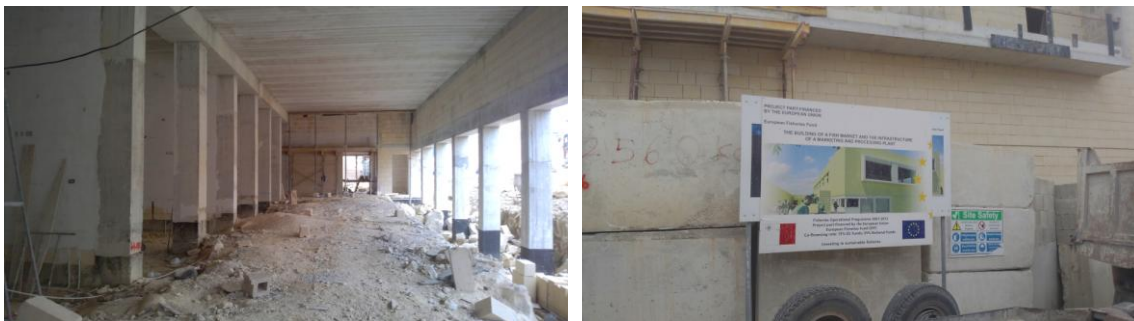
Figure 7: Construction of the New Fish Market
