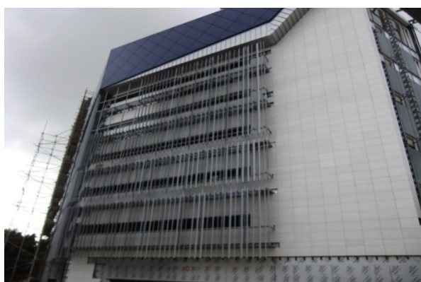
Figure 7 - ERDF199: Ongoing works at the Life Sciences Centre
