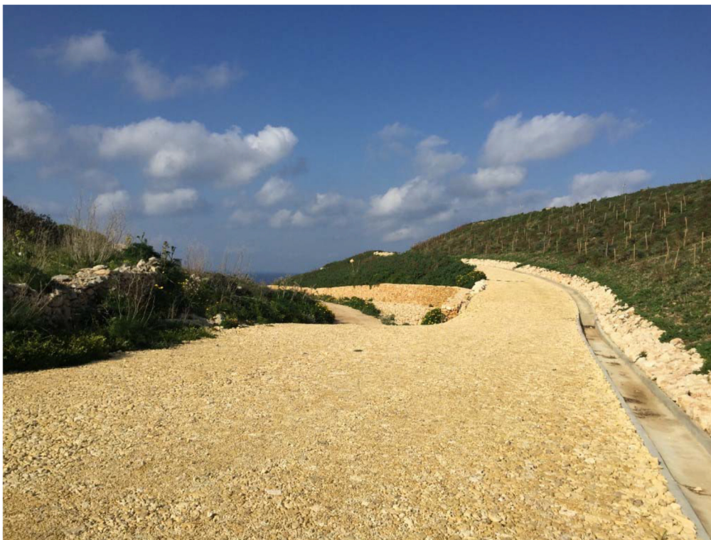
Figure 93 - Qortin - Lower and Upper Access Roads, Landscaping on Slopes, Storm-Water System (gutter and soak-away)
