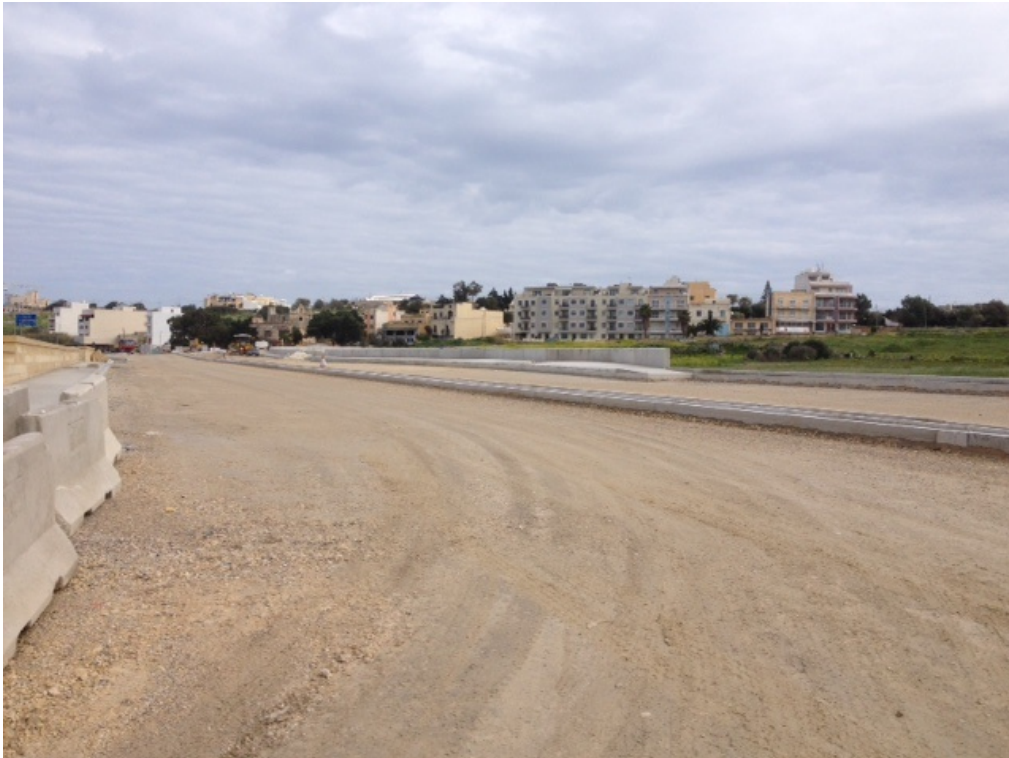
Figure 108 - Phase 1: Road Works leading to the Buġibba Junction
