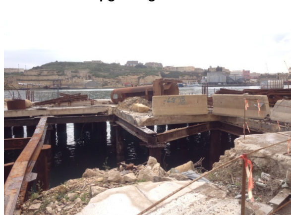
Figure 39 - Quay site – initial phase of upgrading works
