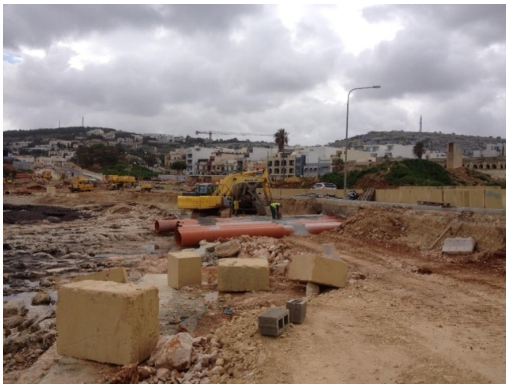
Figure 111 - Phase 2: Installation of Utility Services
