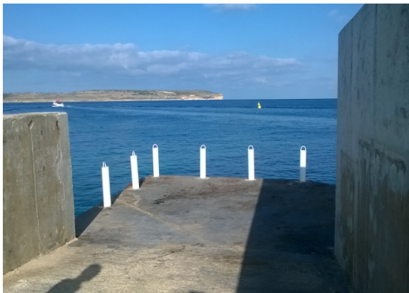
Figure 36 - The Vehicular restraint system at the Ċirkewwa Ferry Terminal
