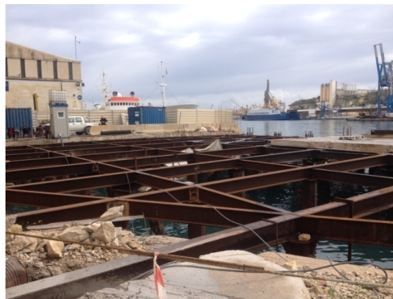
Figure 40 - Quay site - ongoing upgrading works
