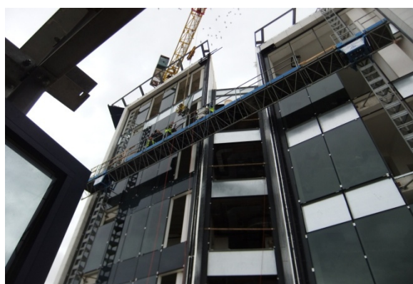
Figure 8 - ERDF199: Ongoing works at the Life Sciences Centre
