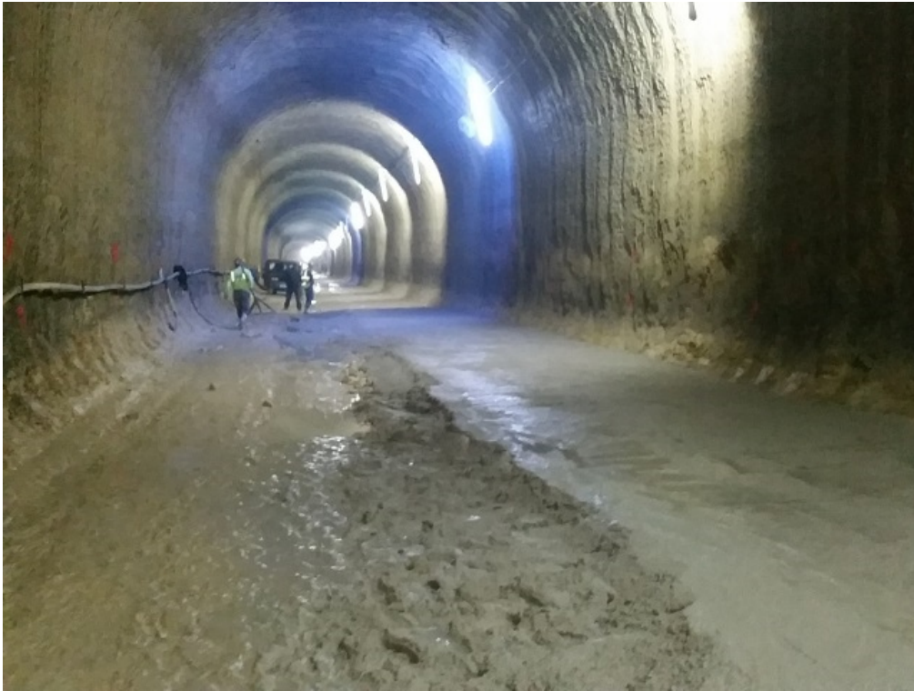
Figure 104 -Birkirkara Trunk 3 Levelling of Floor for Concrete
