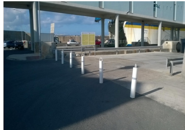
Figure 37 - Safety railings and vehicular restraint system at the Ċirkewwa Ferry Terminal
