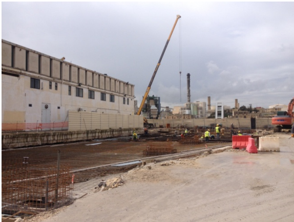
Figure 38 - Ongoing works on the land area behind the shed
