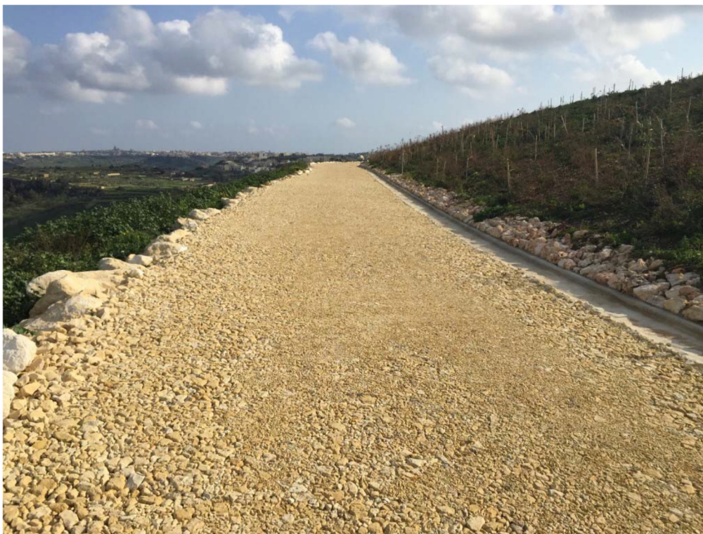
Figure 92 - Qortin - Upper Access Road, Landscaping on Slopes and Storm-Water Gutter
