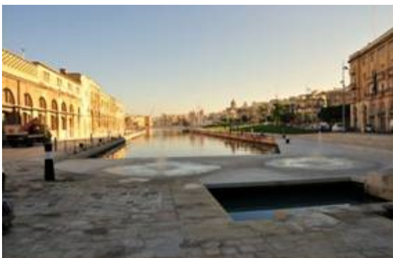
Figure 54 - Rehabilitation and landscaping of Dock head, Cospicua
