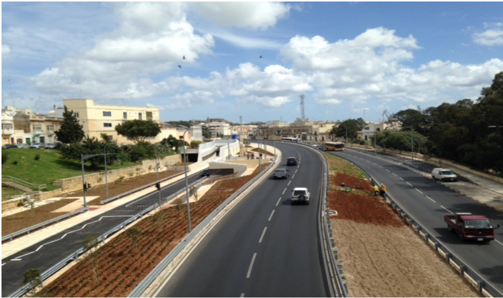
Figure 79 - Marsa Underpass and Diċembru 13 Road
