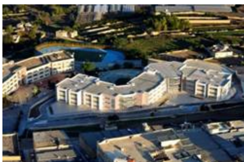
Figure 74 - Gozo College New Boys' Secondary School, Victoria
