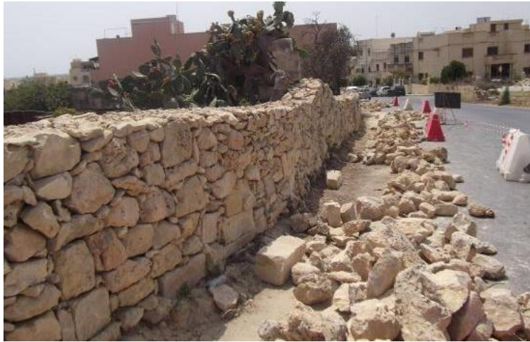
Figure 32 – Restoration of rubble walls under Measure 323
