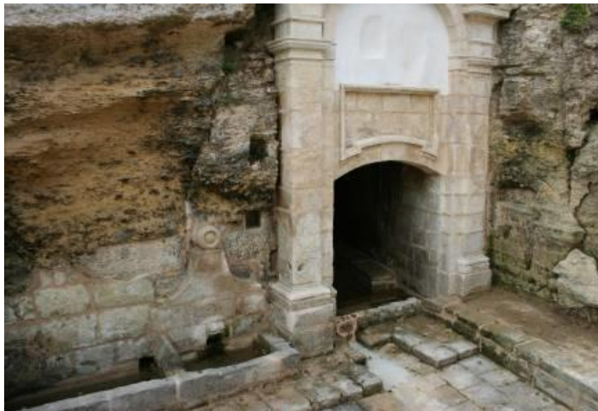
Figure 28 – Restoration works financed under Axis 3
