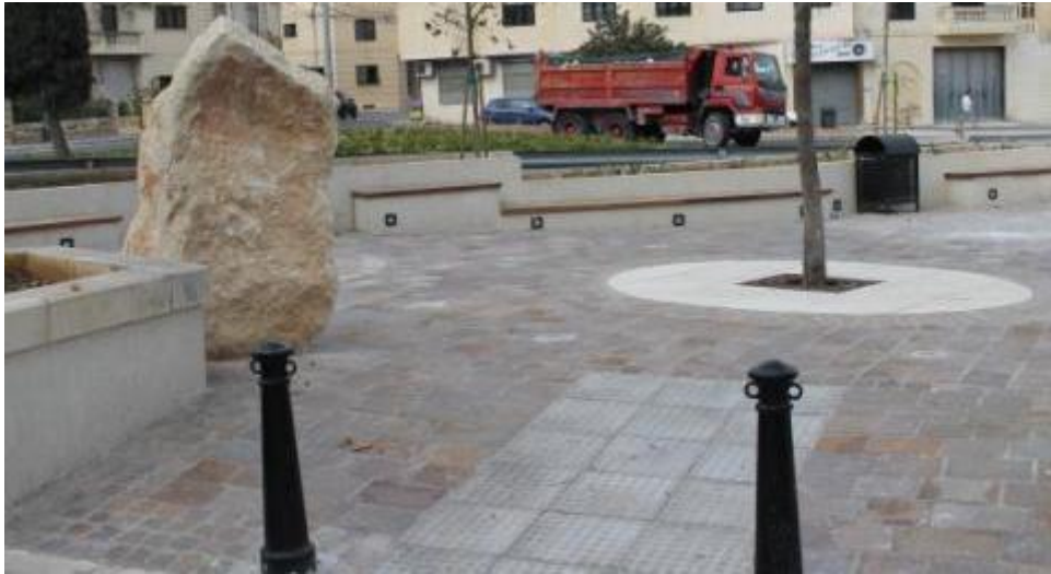
Figure 33 – Works at Mqabba close to finalization
