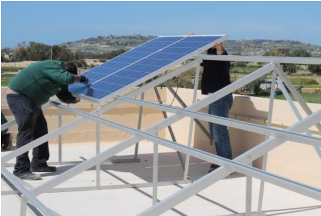
Figure 19 – Photovoltaic panels being installed at a poultry processing plant
