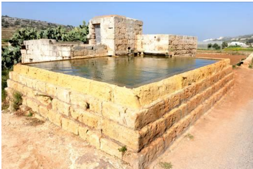
Figure 12 – Several reservoirs were constructed or restored back to working order through Measure 121
