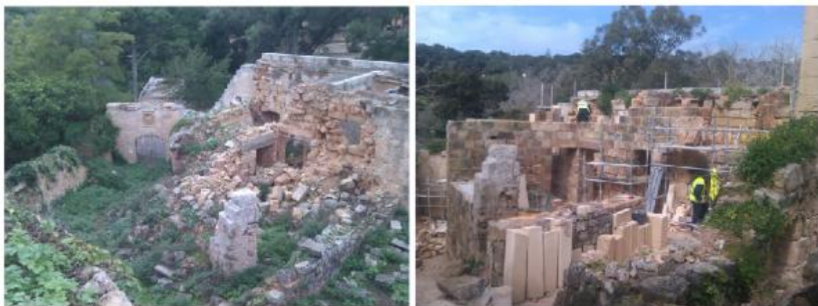
Figure 46 – Restoration works at Razzett tal-Bagħal, Buskett, financed through Measure 323
