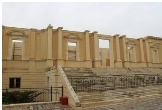
Figure 99 – Construction of a palazzo, M313 project
