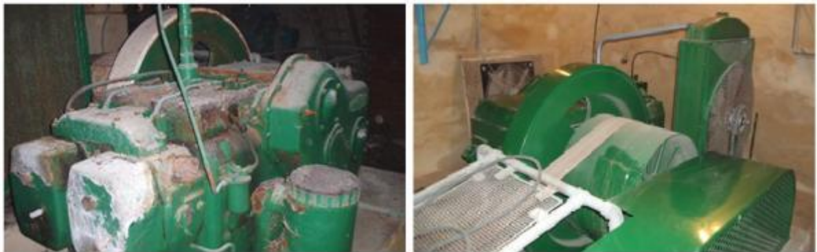
Figure 43 – Restoration of flour mill, M323 project by Munxar Local Council
