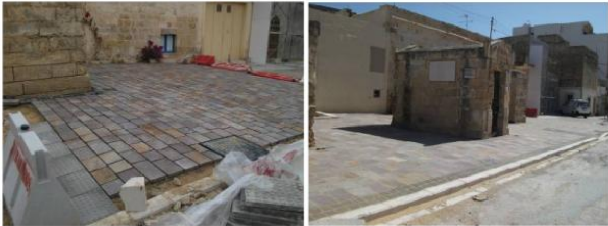
Figure 34 – Works at Mqabba are at an advanced stage of completion
