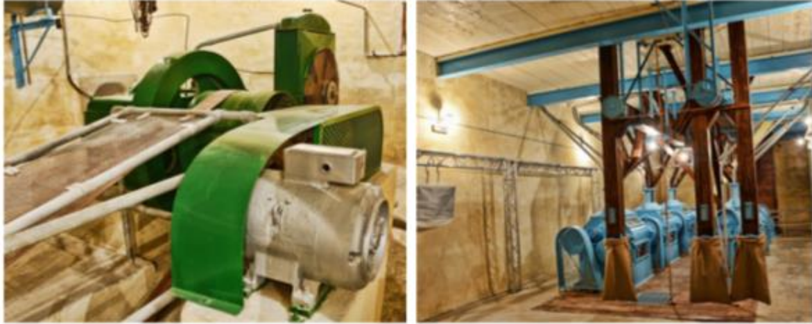
Figure 25 – Munxar M323 project, restoration of flourmill
