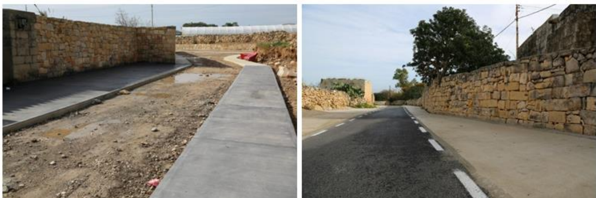
Figure 50 – Rehabilitation of Ta Strejnu area, Zejtun
