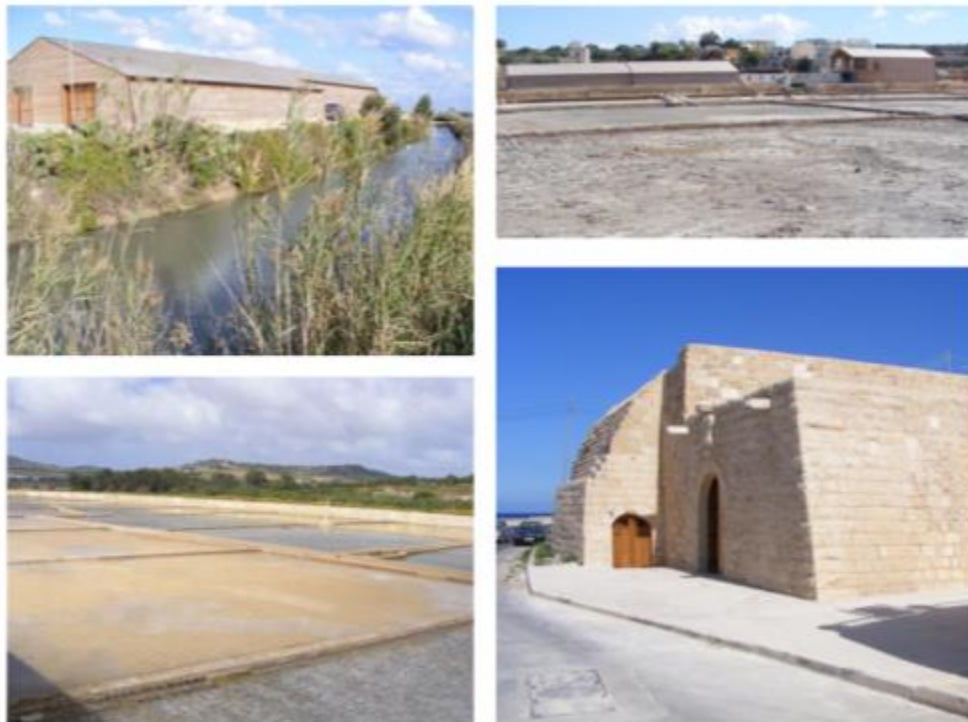
Figure 26 – Storm Water Unit project at Salini Salt pans
