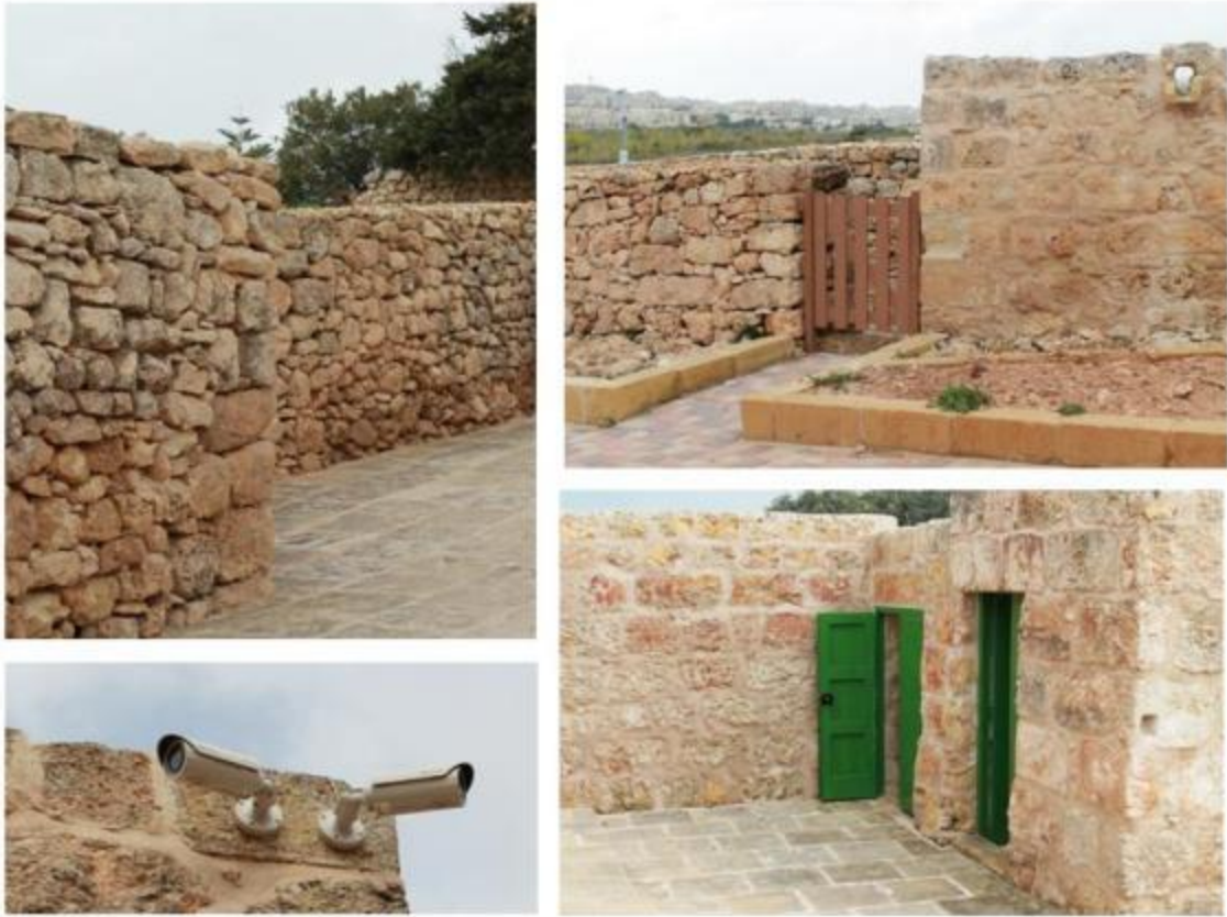
Figure 27 – Mellieha M313/M323 integrated project
