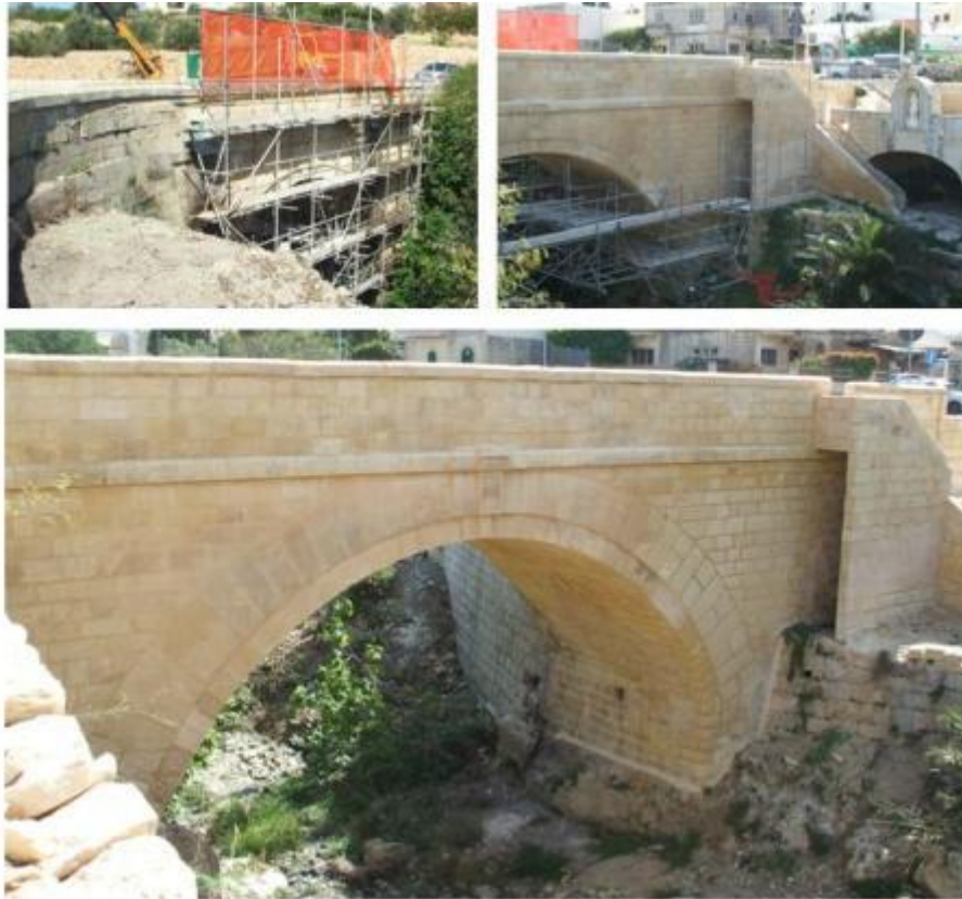
Figure 28 – Restoration of Bridge at Mosta valley
