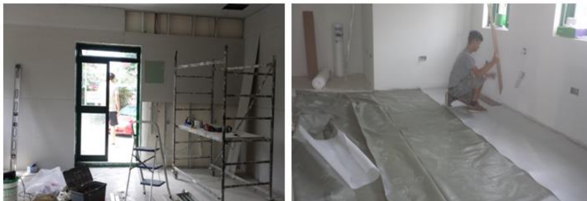
Figure 2 – FASC office refurbishment
