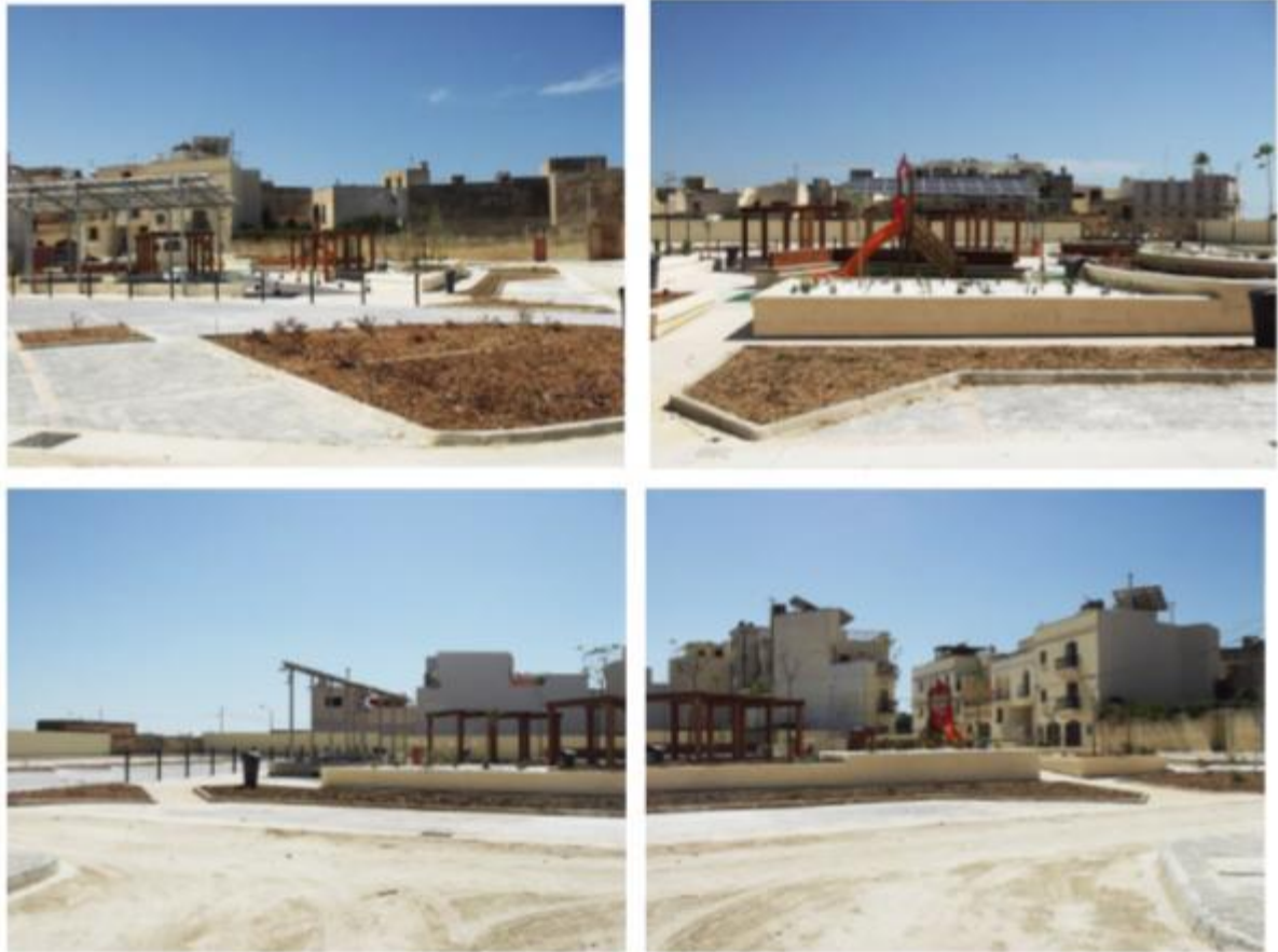
Figure 7 – M313 Kirkop Local Council project
