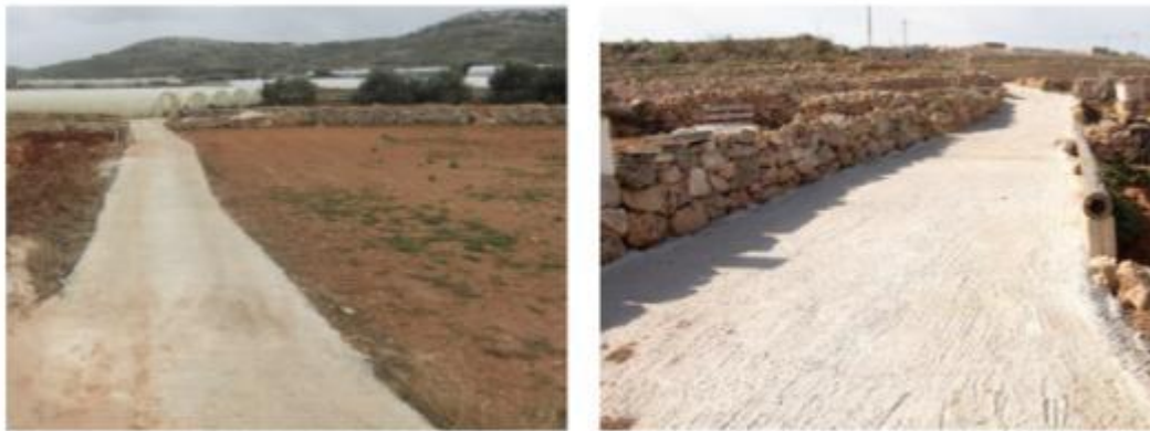
Figure 35 – One of the rural roads which will be resurfaced under Measure 125
