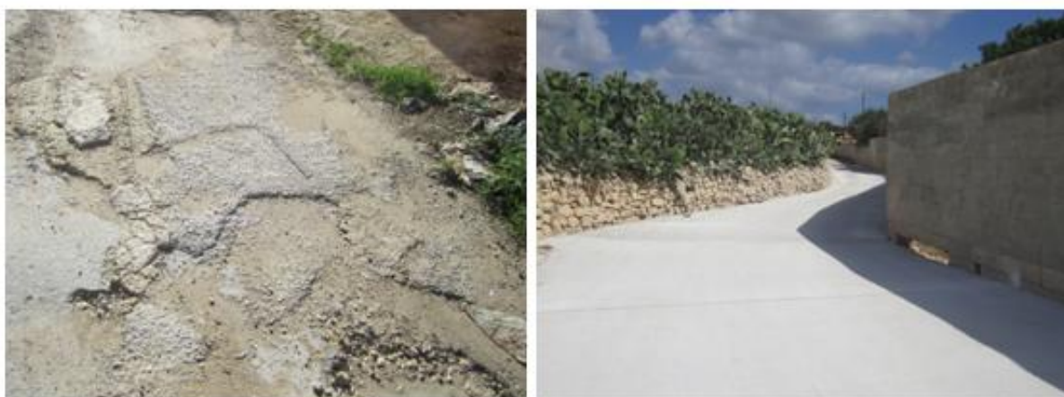
Figure 2 – Road resurfacing by Marsascala Local Council, contracted through GXF
