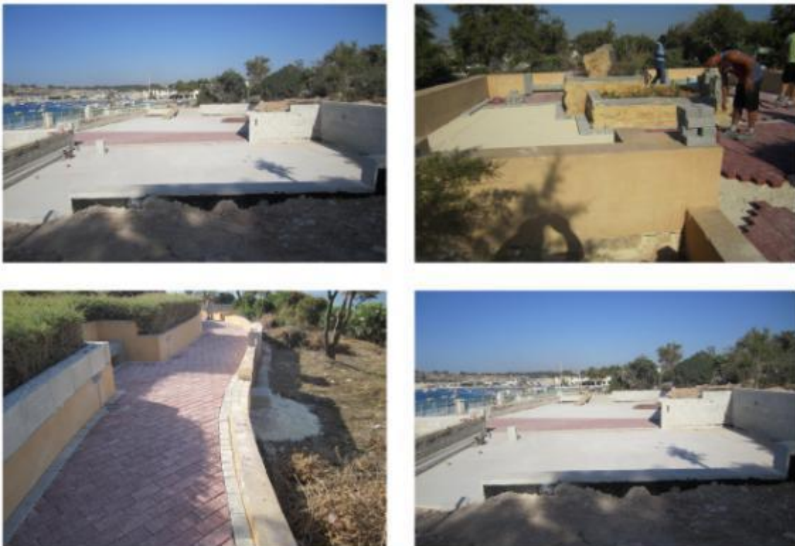
Figure 6 – Marsascalea Local Council project, contracted through GXF
