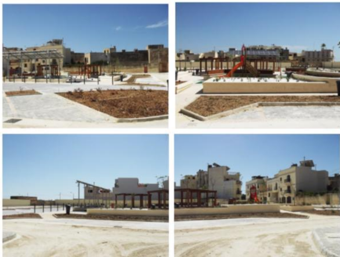
Figure 7 – M313 Kirkop Local Council project
