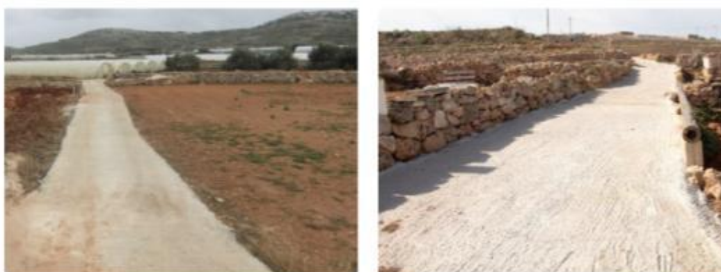
Figure 32 – One of the rural roads which will be resurfaced under Measure 125
