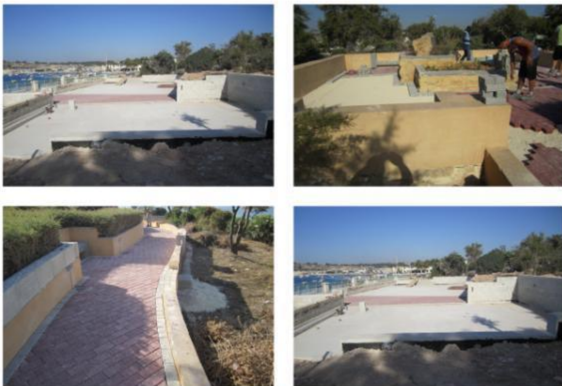
Figure 6 – Marsascalea Local Council project, contracted through GXF
