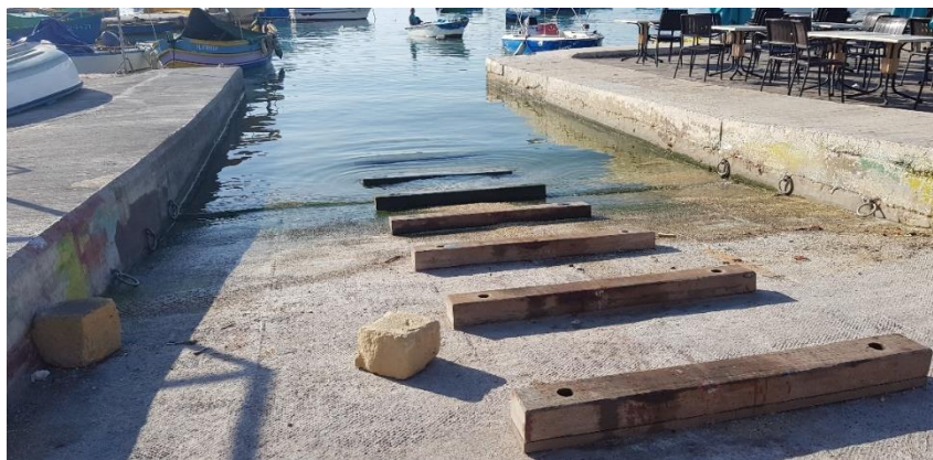
Photo above: An example of finalised works on one slipway.
