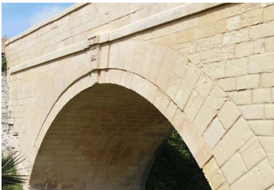
Restoration of bridge in Speranza area, Mosta
