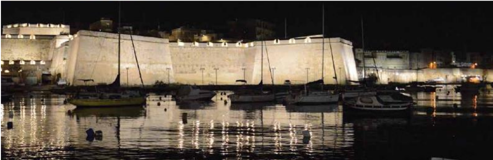
Birgu Lighting System
