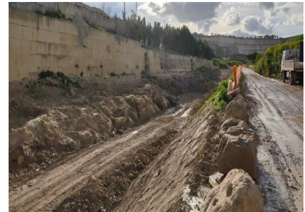
Works on RainWiin project
