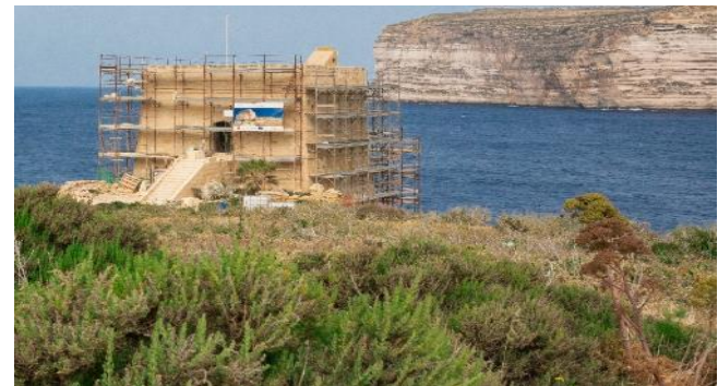
Restoration of Xlendi Tower in Gozo
