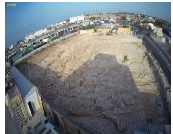
MMRF ongoing excavations
