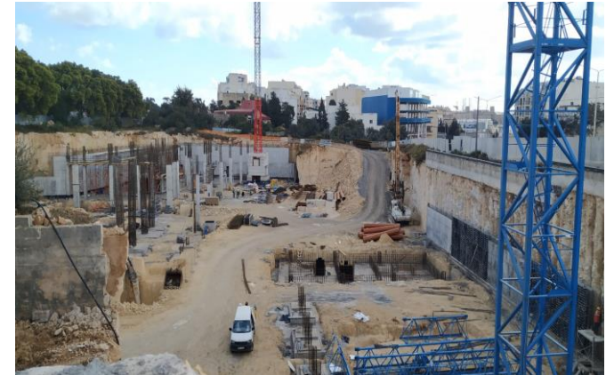
Ongoing construction works on the SLC building
