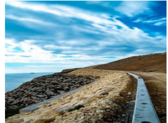
Rehabilitation works at Wied Fulija landfill
