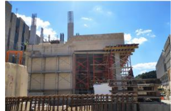
Construction works on TRAKE main building
