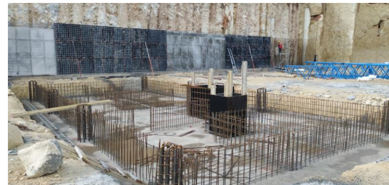
Construction works – core foundation and perimeter wall (SLC)
