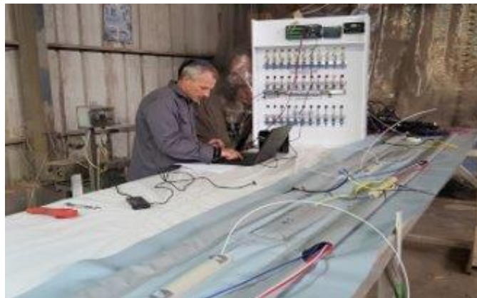
Ongoing preparations for the installation of the water monitoring network
