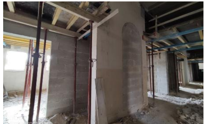
Palliative Care Project – construction works within the Inpatient Unit
