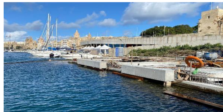
Ongoing works at ferry landing sites in Bormla and Sliema
