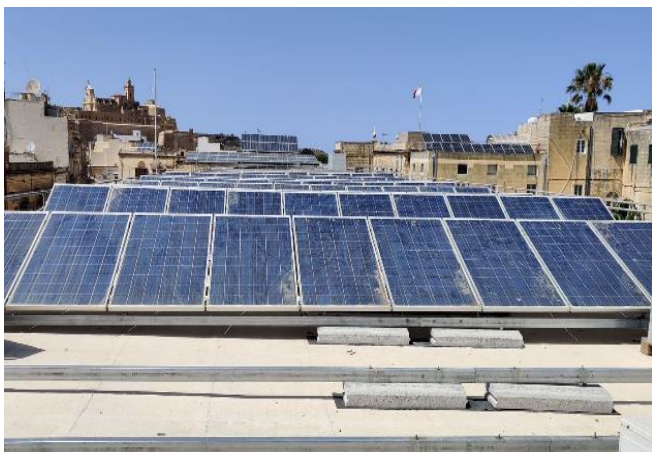
Reinstatement of PV panels at Gozo Administration Centre
