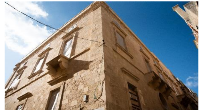
Restoration of a dilapidated building for social housing purposes
