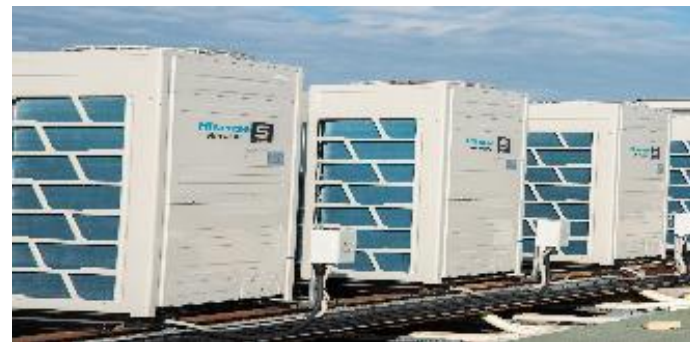
Energy efficiency measures at St Vincent de Paule Elderly People's Home
