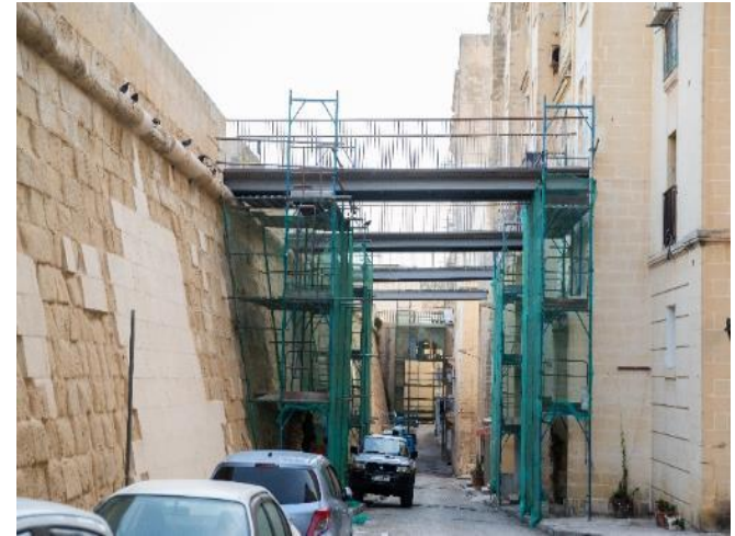
Reconstruction of 5 bridges in Triq il-Funtana.
