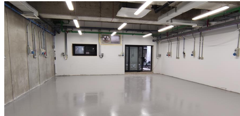
Progress on M&E and Finishes at the Materials Lab (TRAKE)
