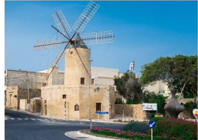
Rehabilitation of windmill in Xewkija, Gozo
