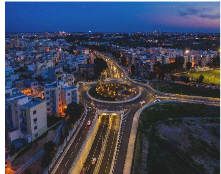
Santa Luċija underpass
