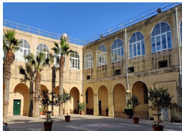
Double-glazed apertures at Gozo Administration Centre
