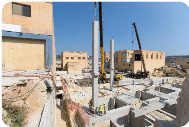
Installation of pillars at Xewkija Enterprise Hub
