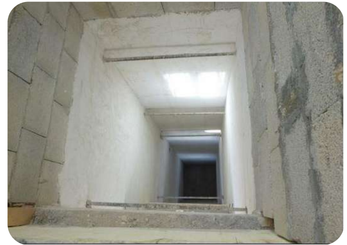
Lift Shaft – Ongoing works for lift installation (Zejtun)
