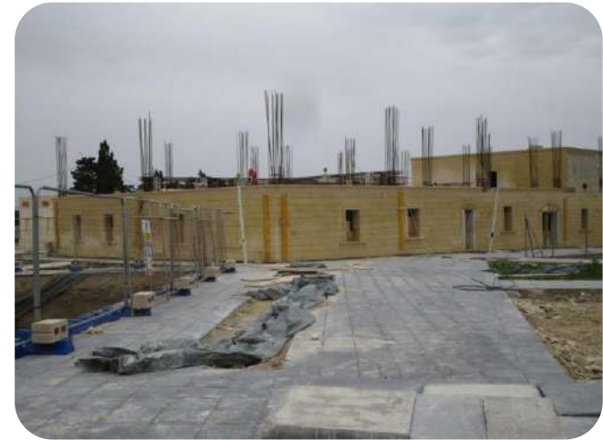
Construction and Landscaping Works at Ta' Qali Crafts Village
