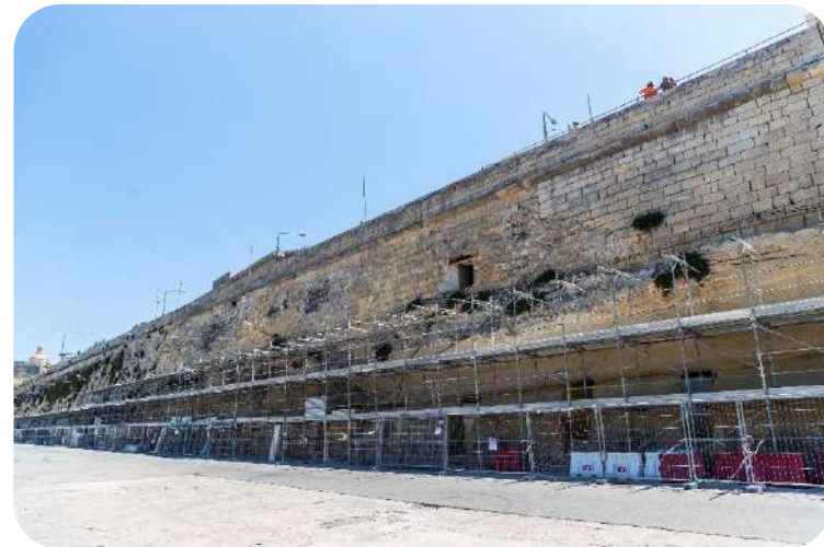
Restoration of common areas in Lower Valletta
