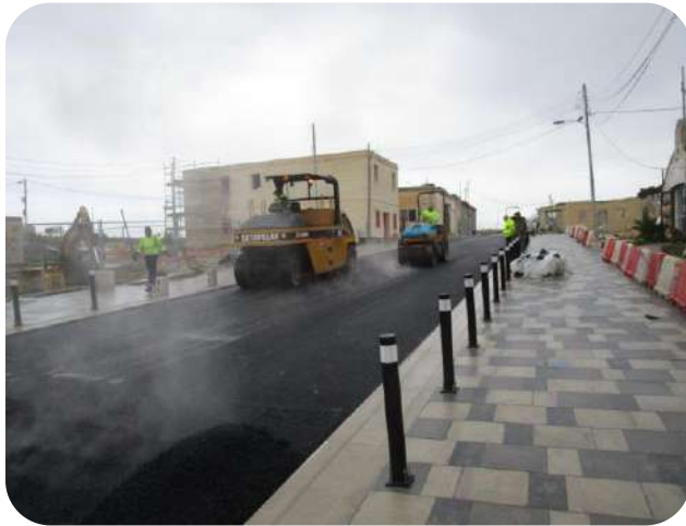
Road Works at Ta' Qali Crafts Village
