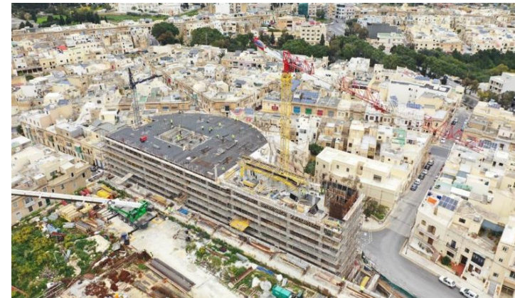
Paola Regional Hub – structural works up to Level 16 almost completed
