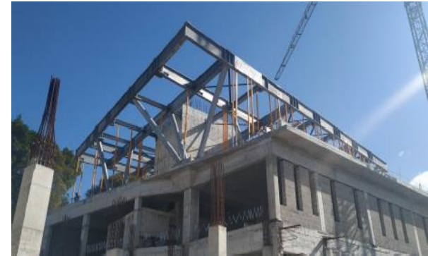
Construction of steel structures at SLC
