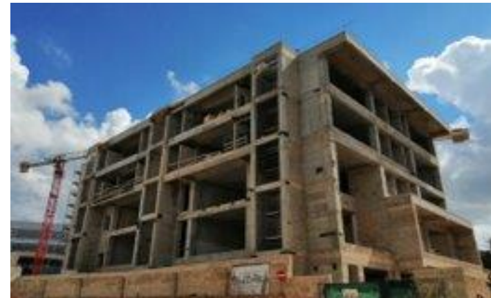
Construction works at an advanced stage at IICT Building
