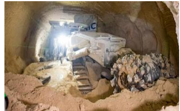
Final breakthrough in Pembroke – Ta' Qali underground tunnel
