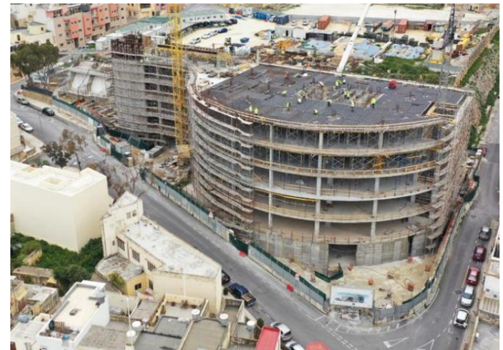
Construction works at Paola Regional Hub Primary Health Care Centre
