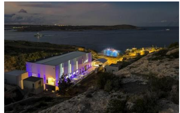
The new Hondoq ir-Rummien RO plant in Gozo
