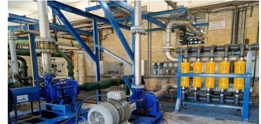
Upgrade of RO under the Major Project
