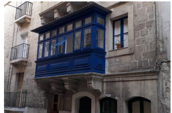
A restored balcony at lower Valletta
