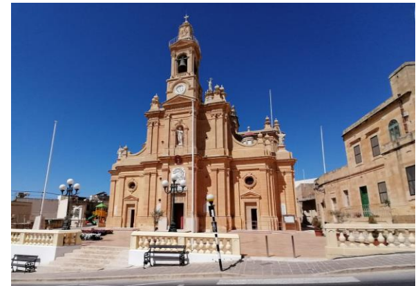
Restoration of the Fontana church façade and parvis
