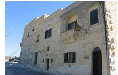
Renewable Energy measures at OASI Foundation – Gozo
