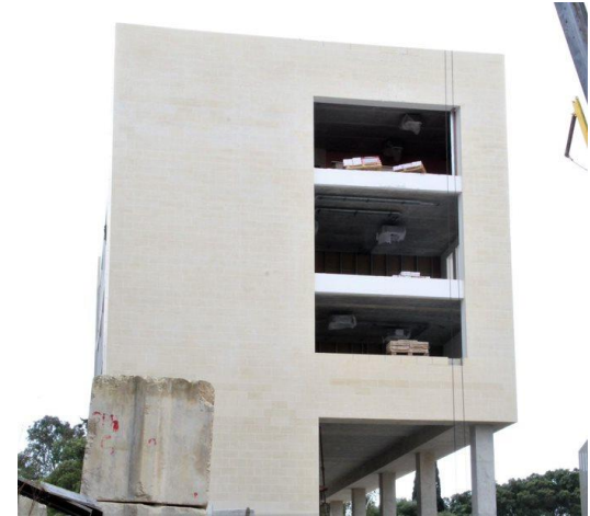
Construction works on the TRAKE main building
