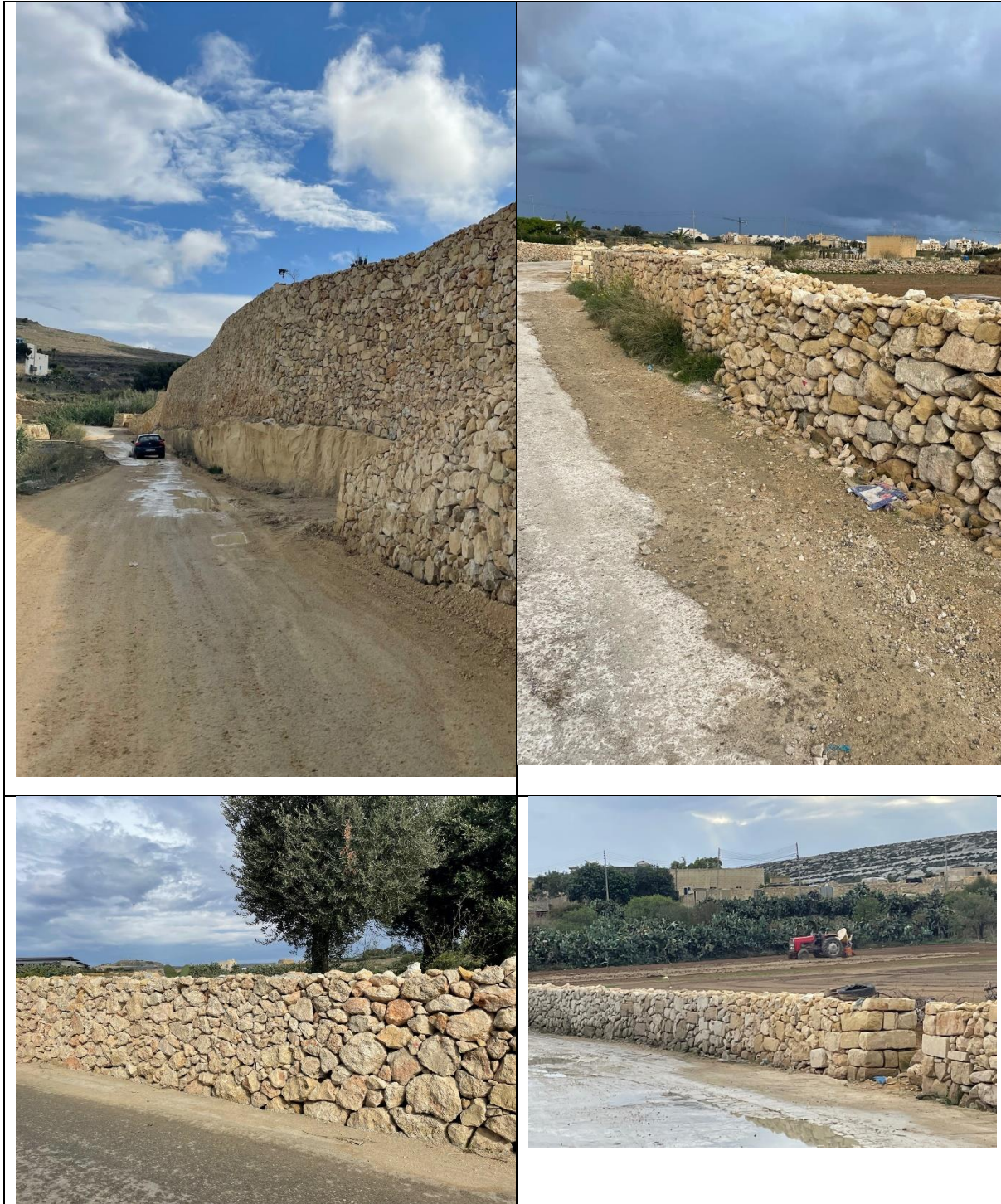
Figure 6.5: Rubble walls in Gozo
