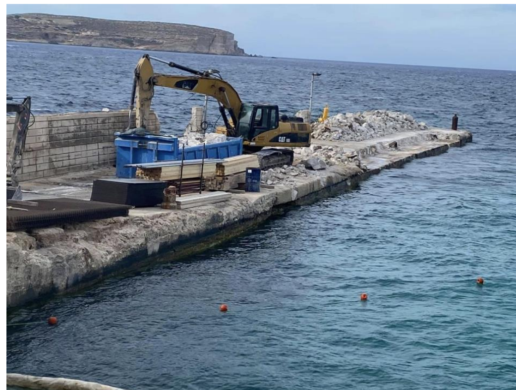
Ongoing works on the Marfa quay
