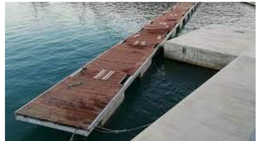
Completed works at Mgarr Gozo
