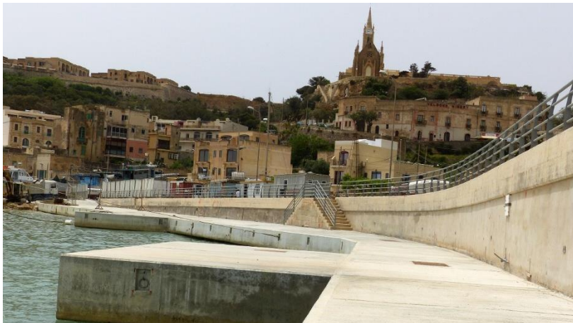
Ongoing works at Mgarr Gozo
