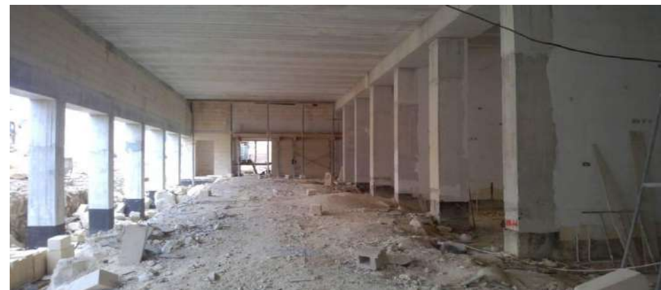
Construction works at the new fish market site, Marsa
