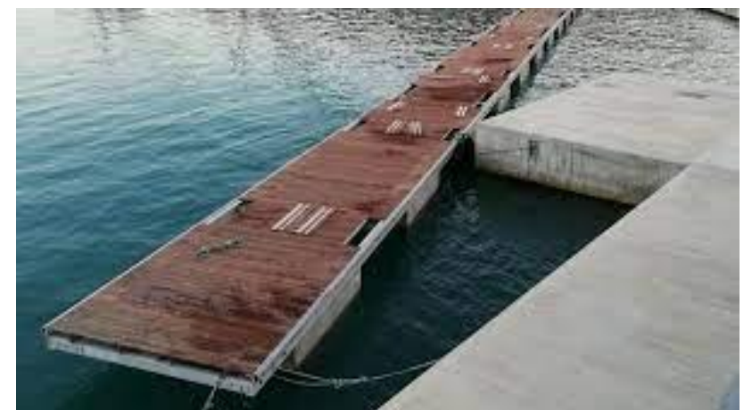
Completed works at Mġarr Gozo
