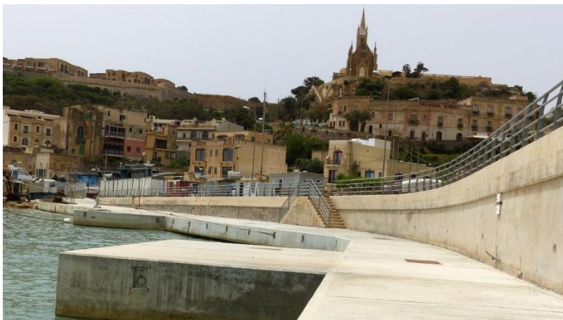
Interim phase works at Mġarr Gozo
