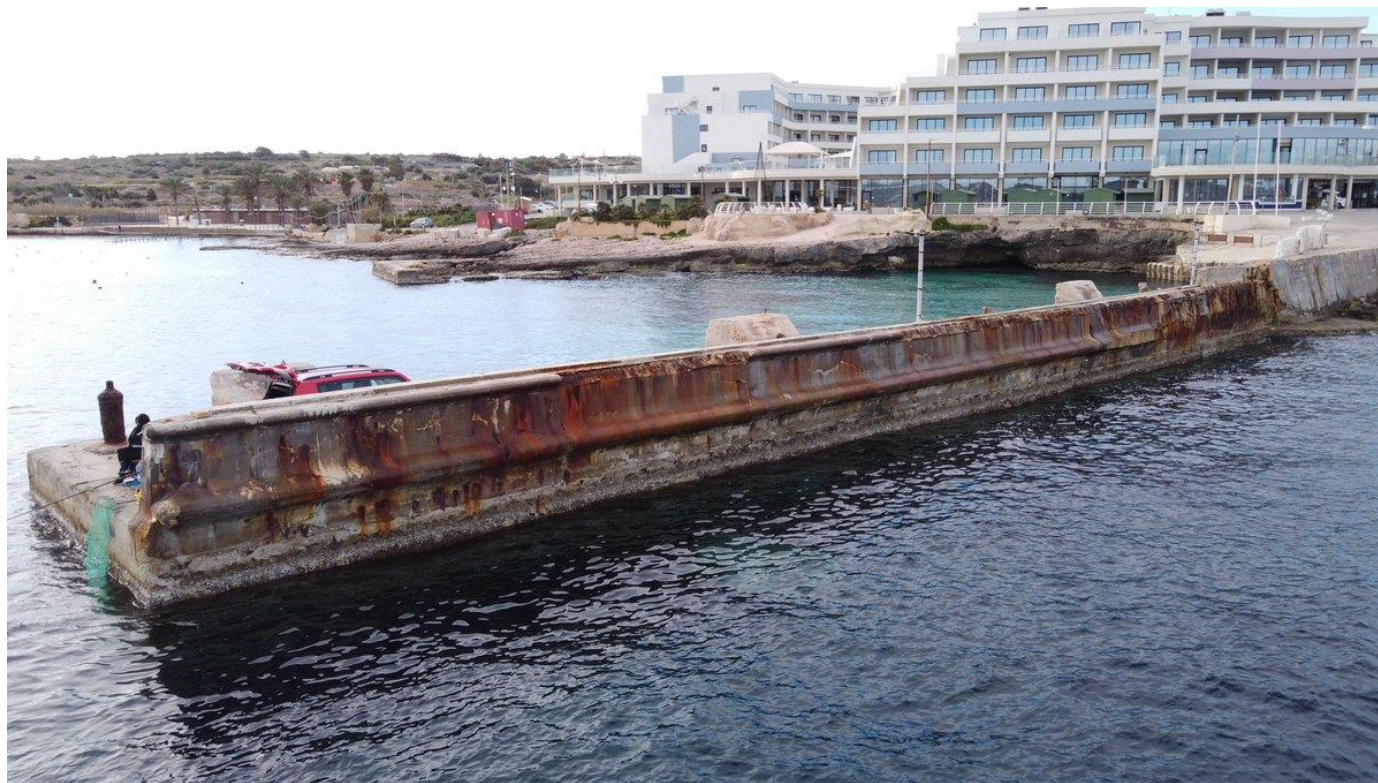
State of the Marfa quay prior to commencement of works
