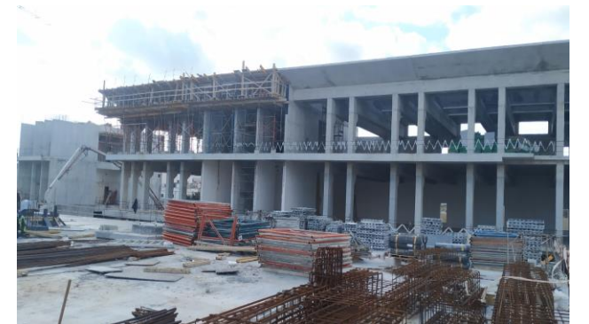
SLC – progress on the various construction zones
