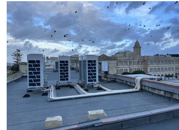
Installation of new EE heating, ventilation, air-conditioning & lighting systems at SVDP
