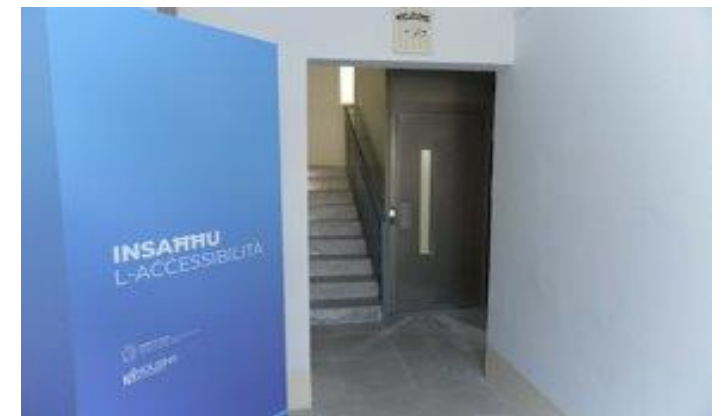
Installation of new lifts at San Gwann Social Housing Estate
