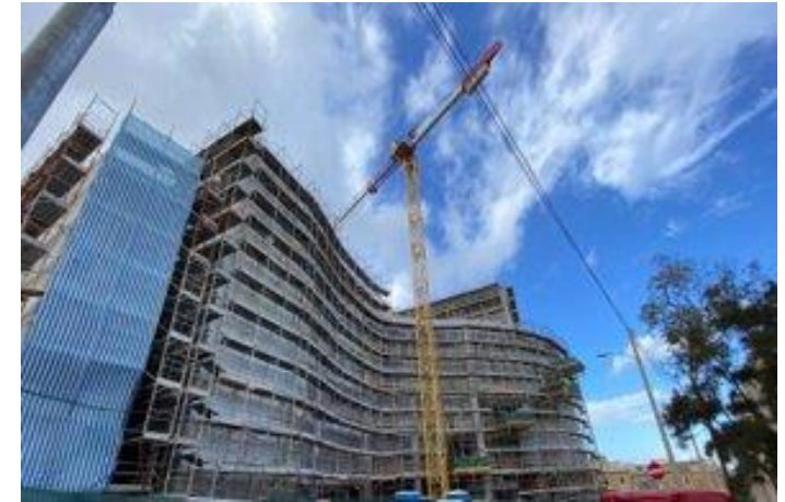
Construction works at Paola Regional Hub Primary Health Care Centre
