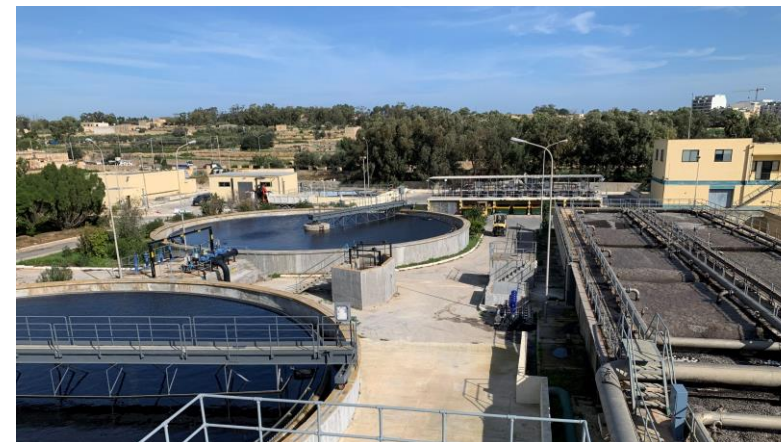
Sant'Antnin Wastewater Treatment Plant
