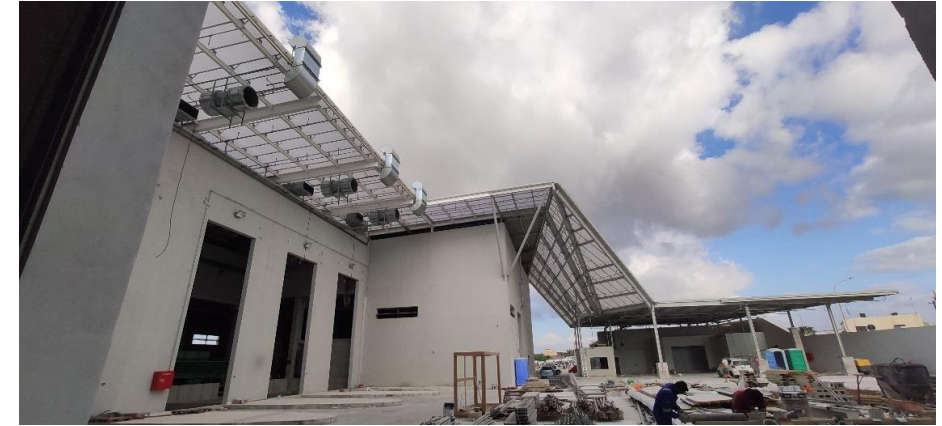
Materials reception area and canopy structure at the MMRF
