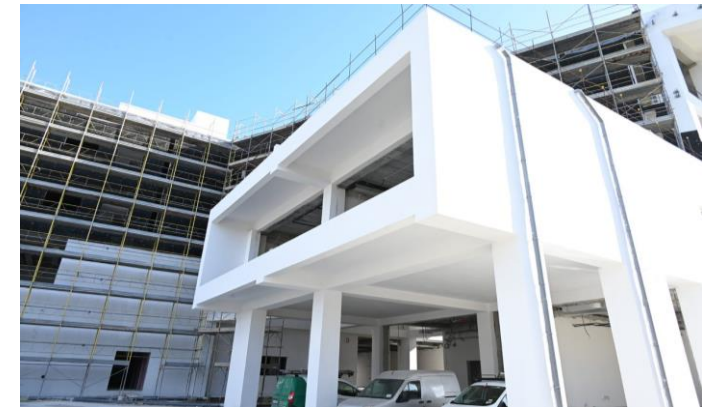
Works ongoing at the MCAST IICT
