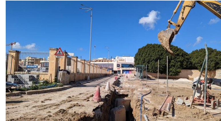
Trenching and pipelaying works in Marsa
