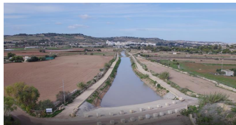
Rainwiin project: Basin 8 – contributing to the increase in overall volumetric capacity
