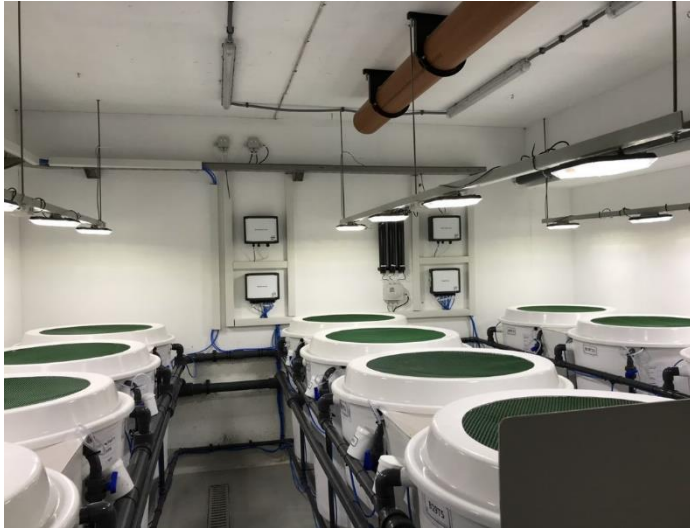
Photo no.1: Lighting equipment.
