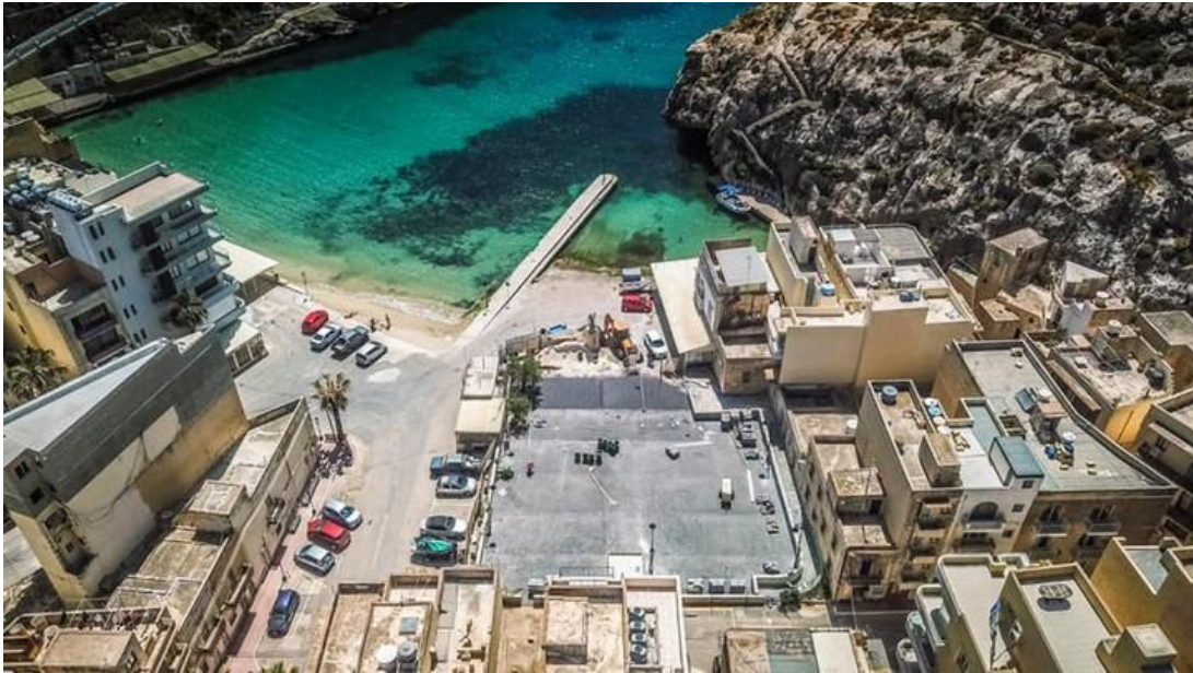
Photos above and below: Works done in Xlendi Gozo
