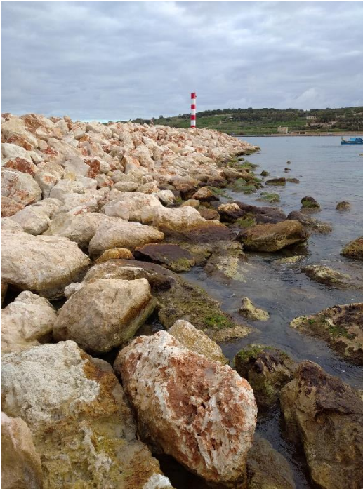
Photo no.1: Outer part of the new breakwater featuring upper coralline limestone quarried from the Rabat-Dingli uplands.
