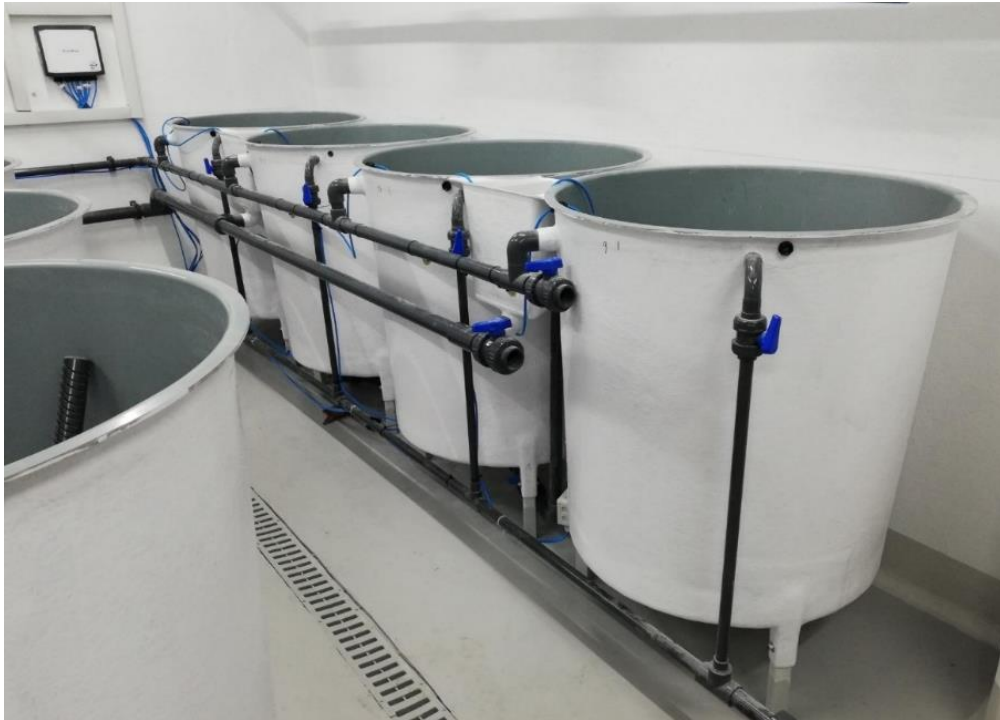
Photo above: New aquaculture tanks with RAS Technology
