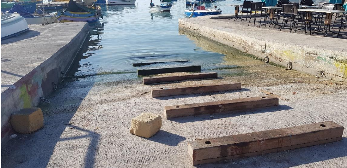
Photo above: one of the refurbished slipway in Marsaxlokk
