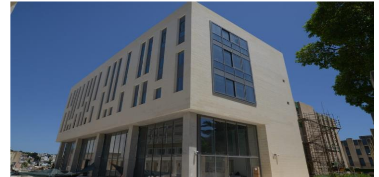
The TRAKE Building at the University of Malta campus
