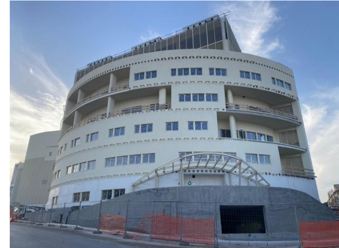
Construction works at Paola Regional Hub Primary Health Care Centre
