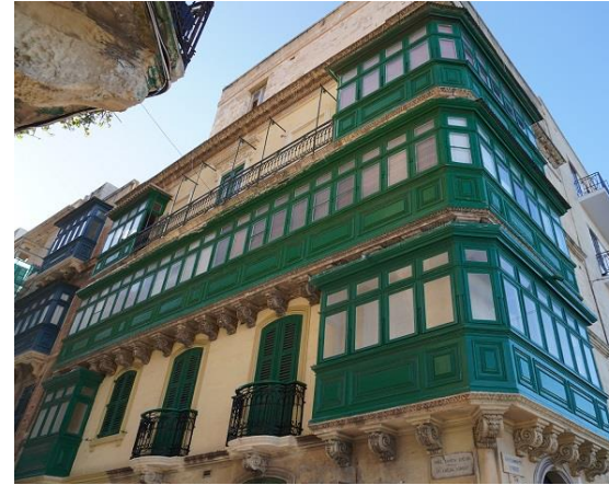
Restoration works for balconies
