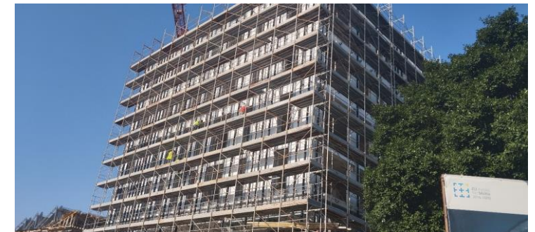
Construction works at SLC site at the University of Malta campus
