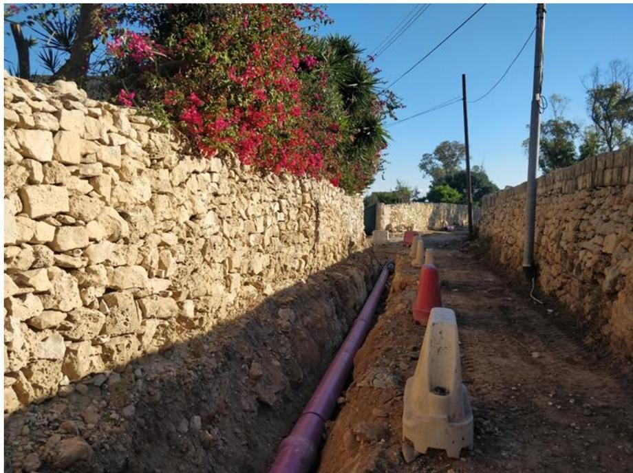
FIGURE 5 - THE SUPPLY OF HIGHLY POLISHED TERTIARY TREATED WATER TO FARMERS, SUPPORTED UNDER MEASURE 4.3 - 'INVESTMENTS IN INFRASTRUCTURE RELATED TO DEVELOPMENT, MODERNISATION OR ADAPTATION OF AGRICULTURE AND FORESTRY'
