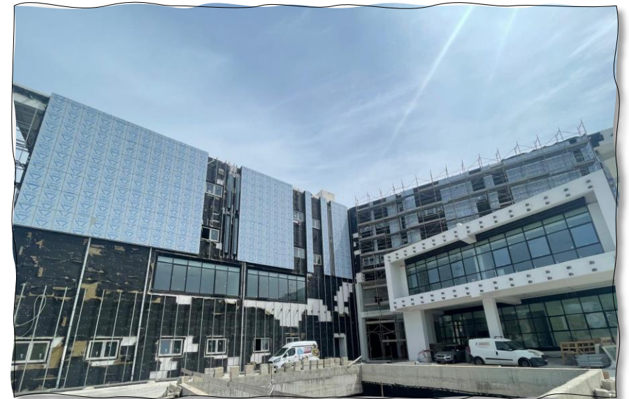
The IICT Institute in its final stages of completion
