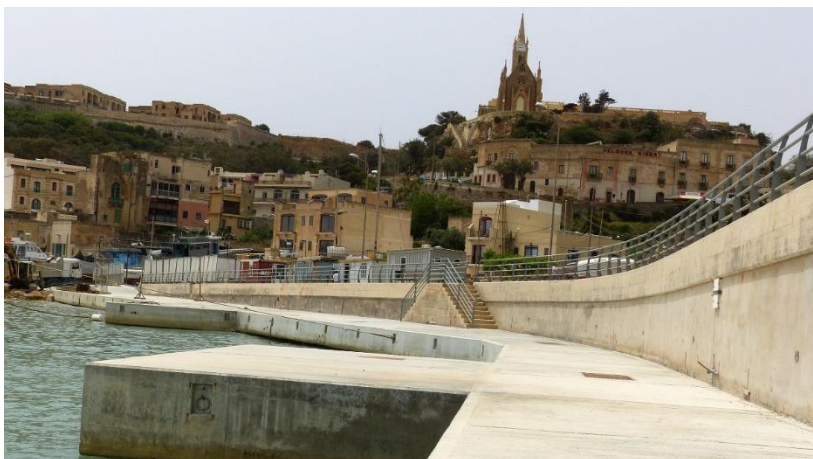
Interim phase works at Mġarr Gozo
