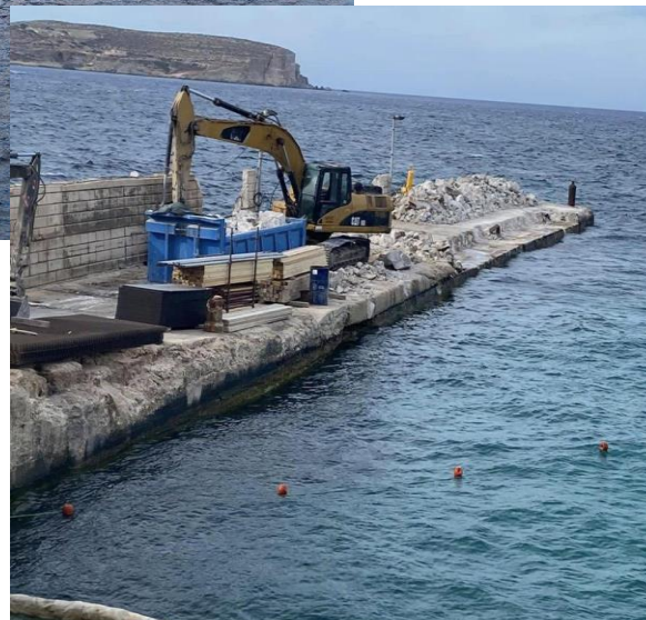
Works on site during the initial component phase
