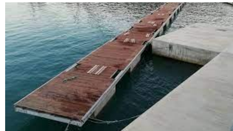
Completed works at Mġarr Gozo
