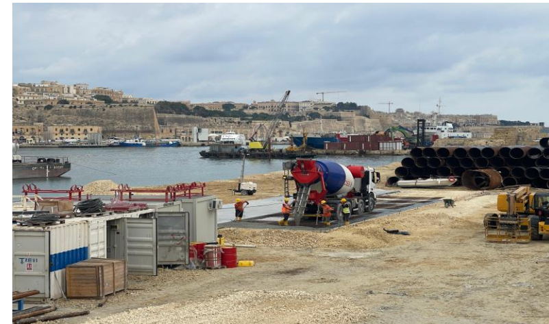
Ongoing Works on site
