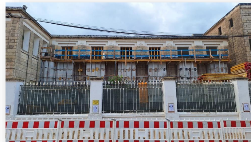
Shoring for the retaining of façade
