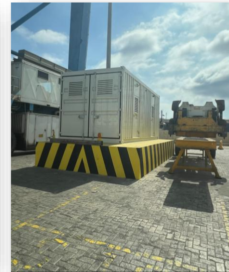
OPS Freeport - Quay Shore Supply selector box
